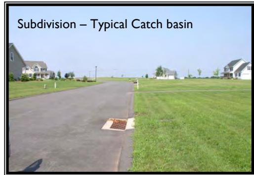
bacteria, sediment, oil, litter and debris. Units need to be maintained routinely and filters need to be replaced on a regular basis to attain maximum removal efficiency. Replacement rates will depend on the type of pollutants being treated, the amount of sediment loading, and the regularity of street sweeping. Estimates for the cost of inserts range from \$650 per filter to \$1,300 per filter. Cost for inserts that targeted bacteria in a pilot project in Norwalk, CT ranged from \$800 - \$1,000.
