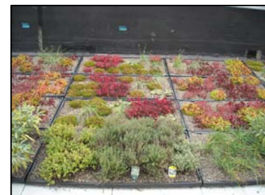
The Hollander Foundation Building green roof in Hartford
