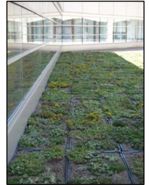
Gant Plaza green roof at UConn - Storrs
