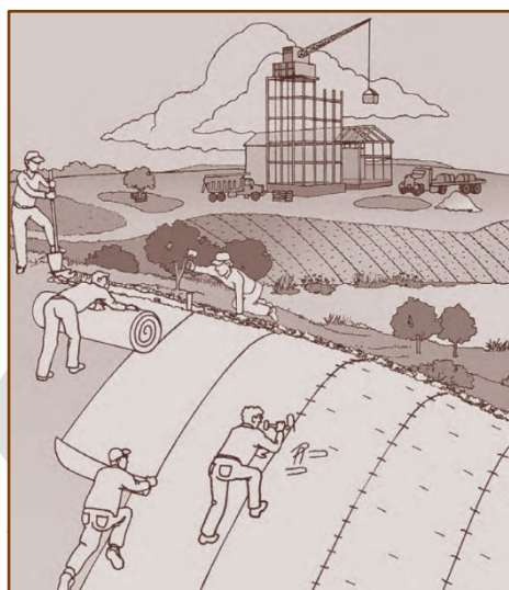
Figure 5- 13 Example of Temporary Erosion Control Blanket Installation
