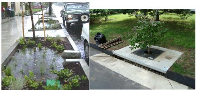
Figure 3.10 – Examples of planter box designs in high density development in Connecticut.
