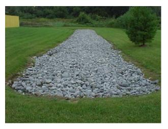
Figure 4.28 – Infiltration trench. Source: Connecticut Department of Environmental Protection.
