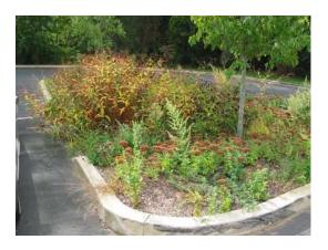
Figure 4.13 – Bioretention in use as a parking lot island in Branford, CT. Source: Connecticut Department of Environmental Protection.
