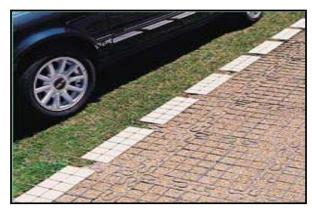
Figure 4.15 – Permeable pavement. Source: Connecticut, 2004.
