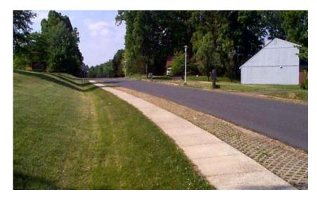
Figure 3.5 - Narrow low-volume road section with sidewalks, shallow swale and porous pavement shoulders.
