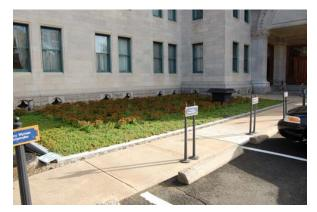
Figure 3.13 – Bioretention retrofit.
