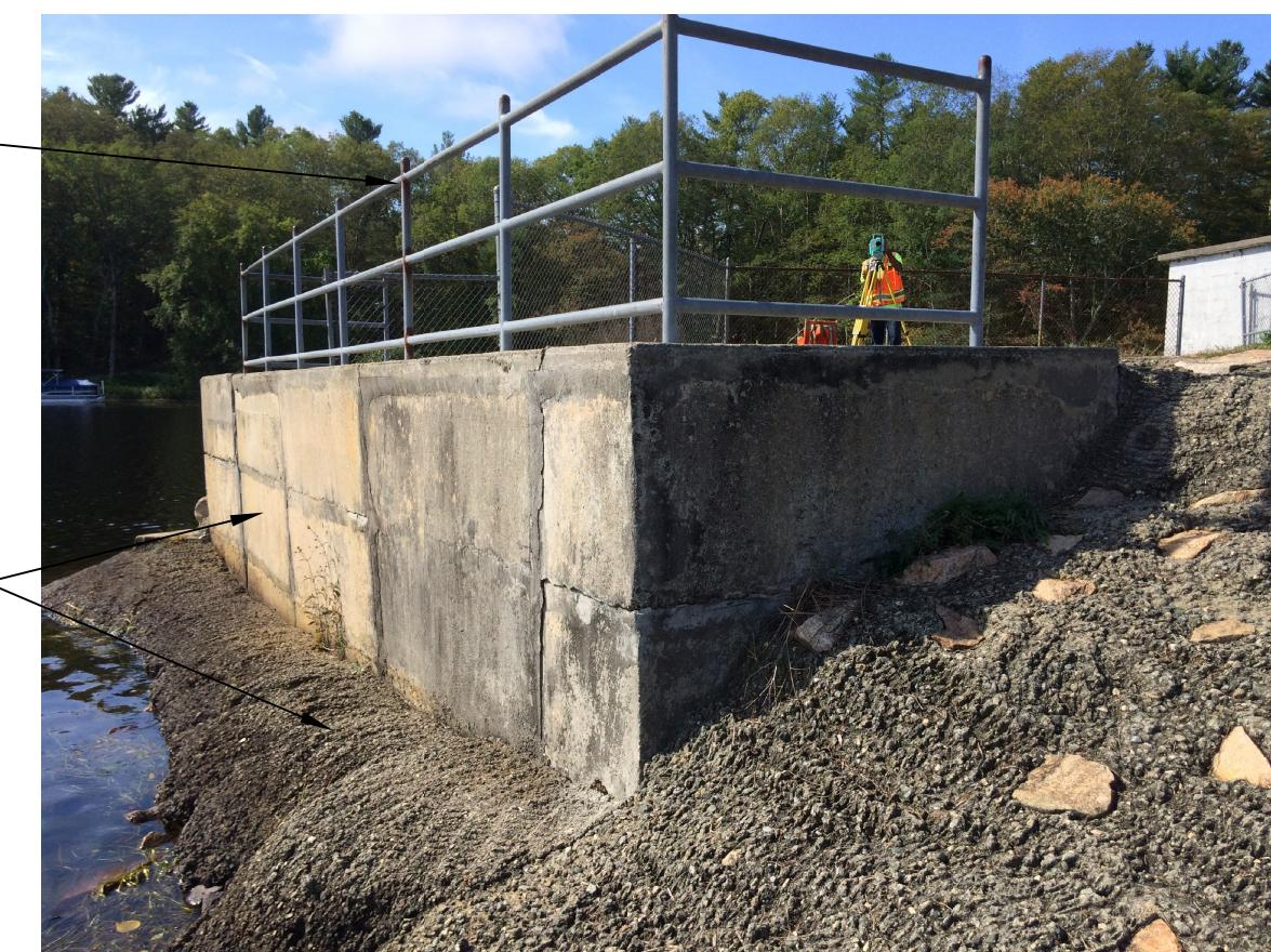
REMOVE AND DISPOSE OF ALL CONCRETE PORTIONS OF PLATFORM, INCLUDING CONCRETE SPLASHED RIPRAP.
