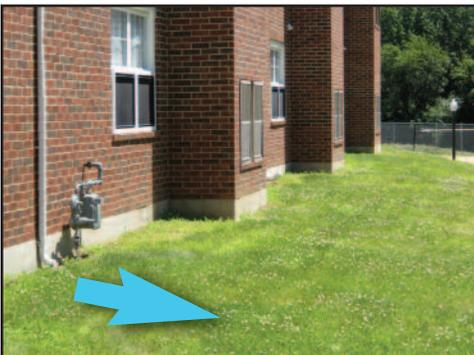
An important distinction when dealing with impervious cover is whether it is *connected* or *disconnected*. (Top image) A parking lot which is directly connected to the drainage system, which flows into a nearby stream. (Bottom image) Runoff from the impervious rooftop is channeled via the leader into an extensive lawn area where the water can infiltrate, effectively disconnecting this portion of the roof from the drainage system.
