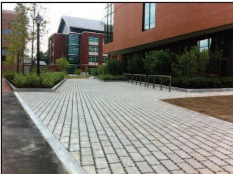
Examples of stormwater practices, drawn from the UConn campus in the Eagleville Brook watershed. (Top) Permeable asphalt parking lot during a rainstorm, showing water running off adjacent conventional asphalt drive but infiltrating into parking lot. (Bottom) Walkway made of concrete paver blocks set so that water can infiltrate between the blocks.
