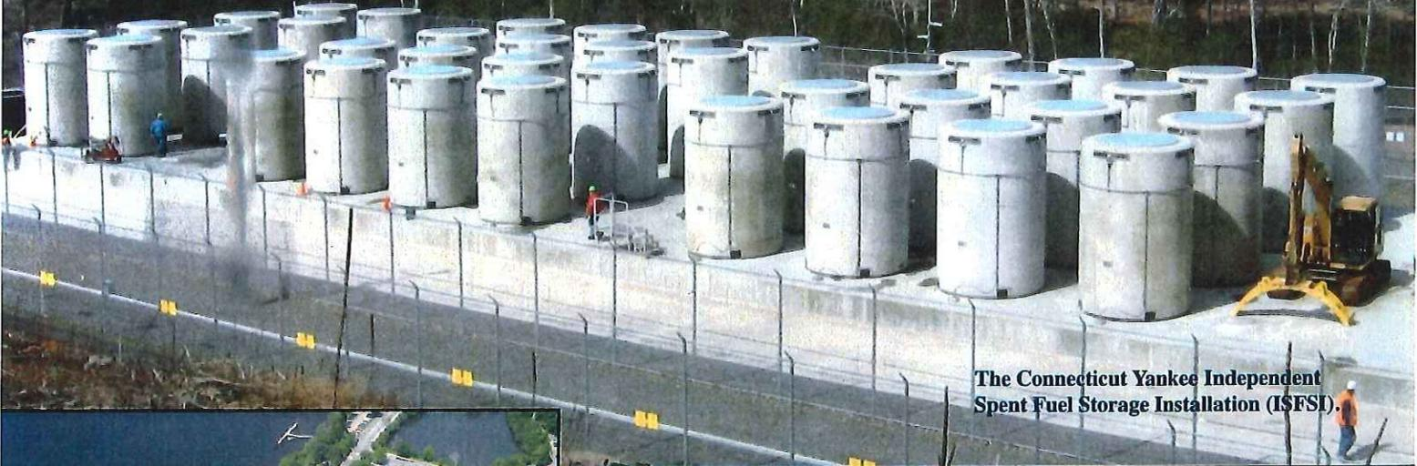
The Connecticut Yankee Independent Spent Fuel Storage Installation (ISFSI).
