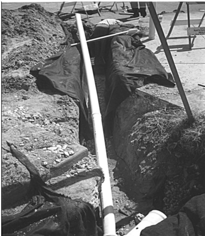
Figure 6.2. Installing an underdrain
