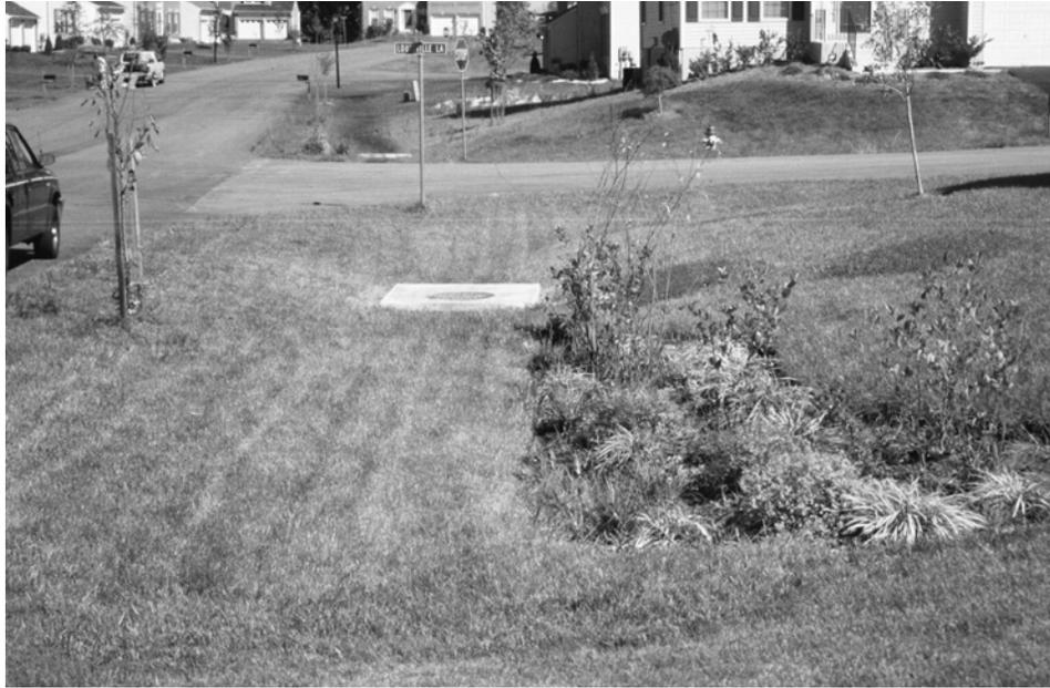
Figure 2.5. Swale-side bioretention
