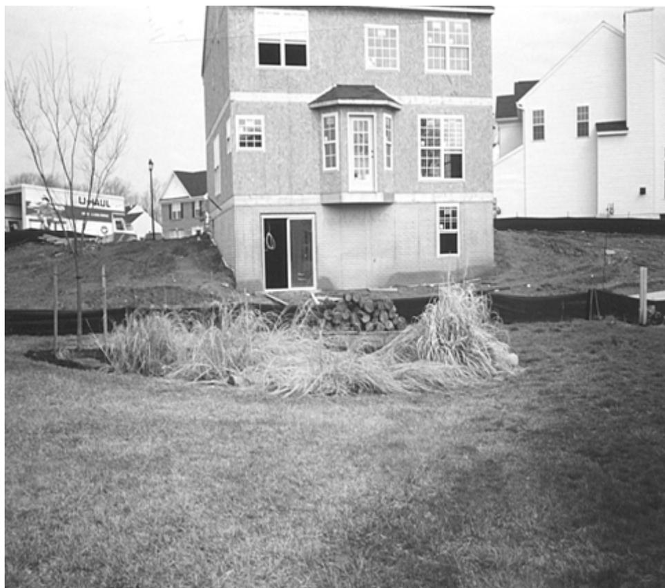
**Figure 6.1.** Silt fence around bioretention
