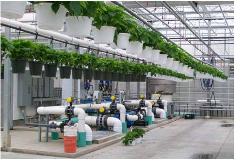
Geremia Greenhouses uses flooding floors and a drip irrigation system to conserve and reuse water.
