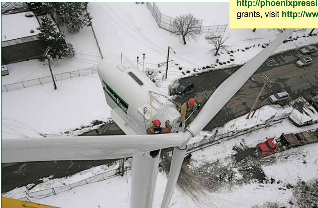
Installing Gus(t), the Phoenix Press wind turbine.
