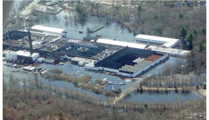
The average National Flood Insurance Program (NFIP) non-residential flood claim is almost $90,000. Photo courtesy of The New London Day .
