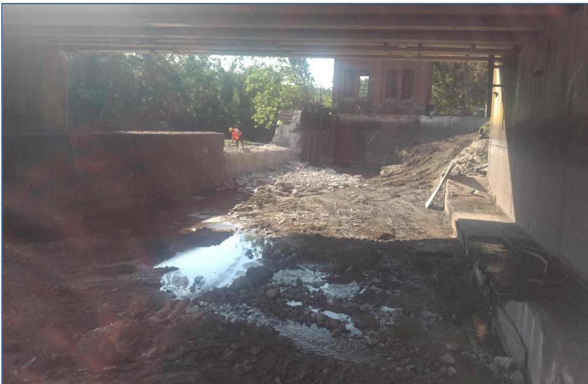
*The view of the Upper Collinsville power canal from under the Route 179 bridge looking downstream to the brick powerhouse. Both this power canal and the tailrace have been de-watered with cofferdams and years of deposited sediment has been excavated. The notch in the dam will host adjustable crest gates that will replace the wooden flashboards that used to be on the dam. The future fishway will pass under the bridge on the far right side.*
