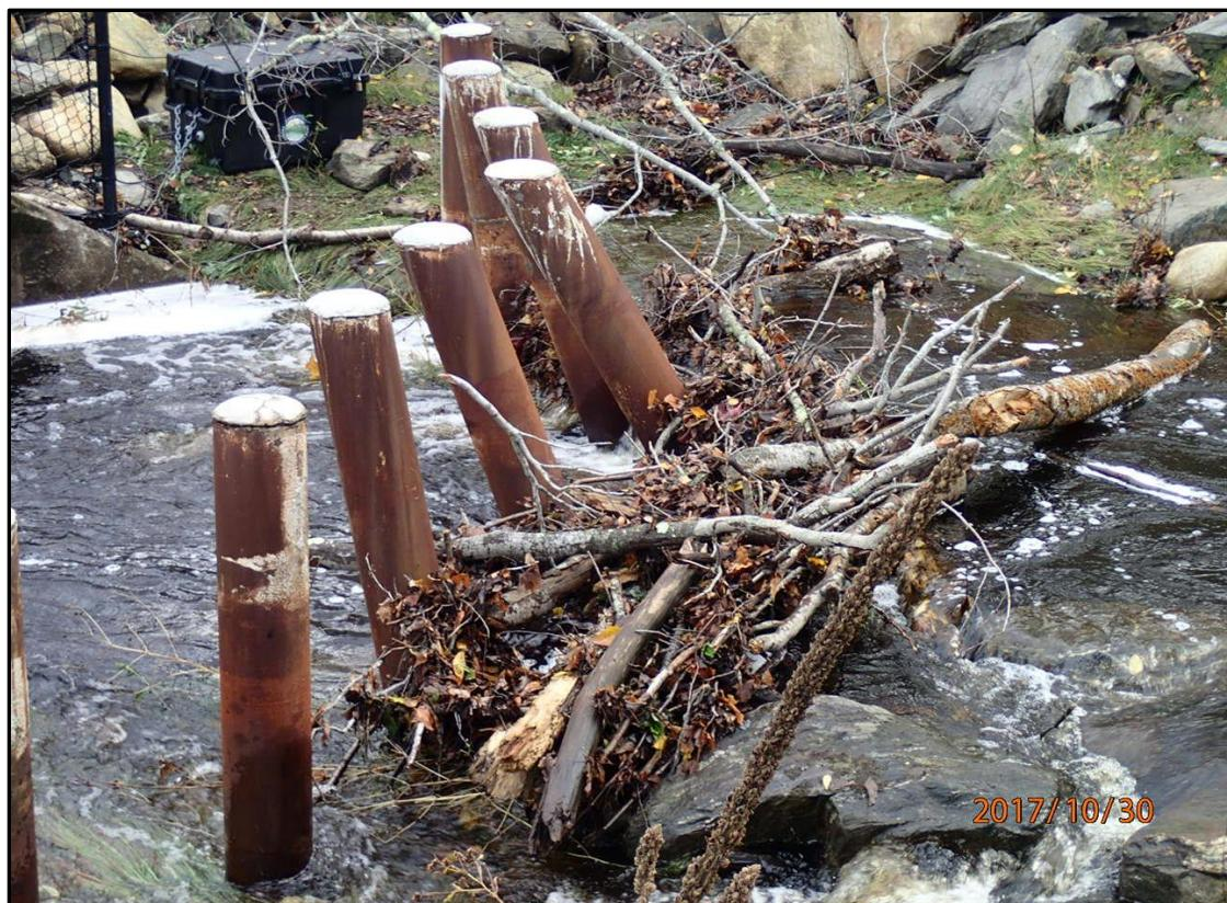
**Figure 30. Accumulation of smaller woody debris on secondary rebar trash rack after October 2017 storm event.**
