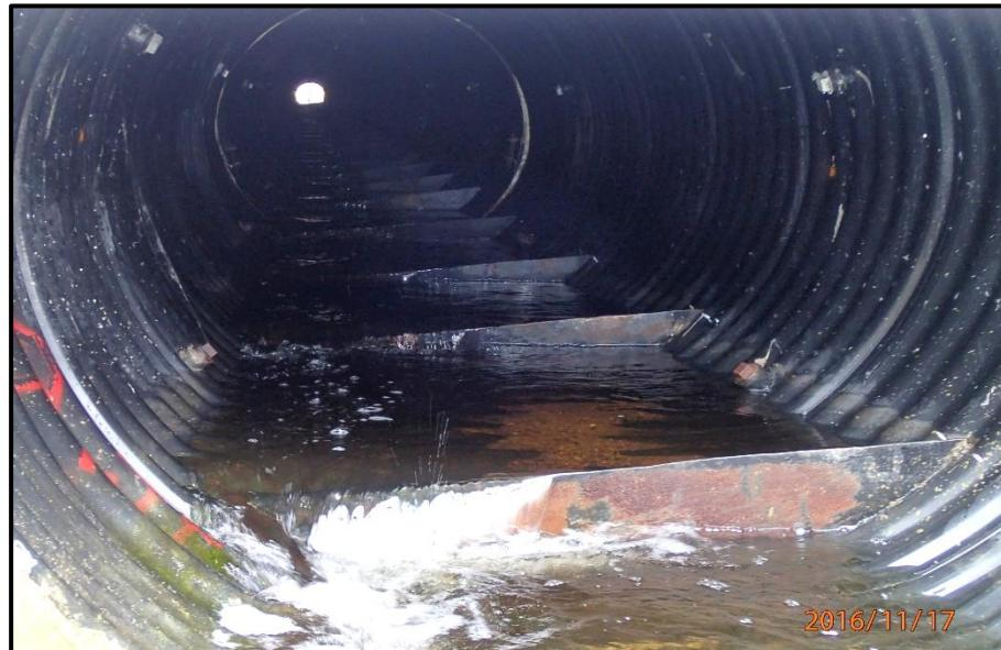
**Figure 5. View of primary inlet trashrack and collection of woody debris after storm event.**
