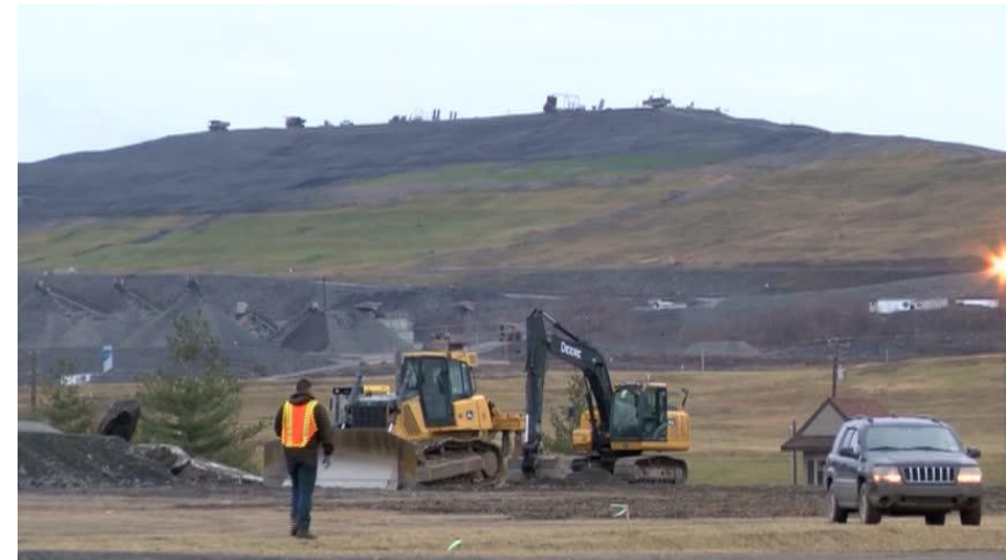
Keystone Sanitary Landfill, PA, managed approx. 180,000 tons of CT MSW in 2022
