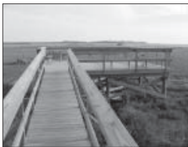
Completed observation platform offers view of Clinton Harbor.
