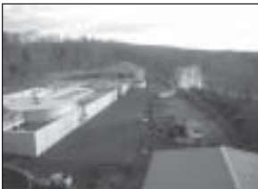
Jewett City treatment plant treats CSOs
