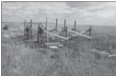
Wildlife observation platform, Hammonasset Beach State Park, Madison, under construction by State Parks Div. staff. Elevated platform protects underlying tidal wetland vegetation.
