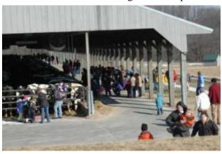
The design of the Chesmers' free stall barn has adapted their Graywall Farms dairy operation to high temperatures by maximizing natural ventilation which keeps the cows cool enough to produce milk.
