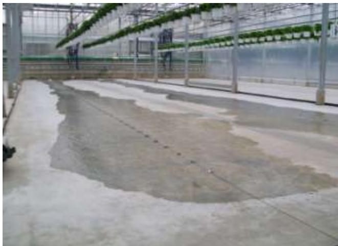
*Flooding floor plant irrigation systems are more efficient than traditional, overhead watering, and reduce plant susceptibility to pests and diseases.* (Photo Credit: CT DEEP)
