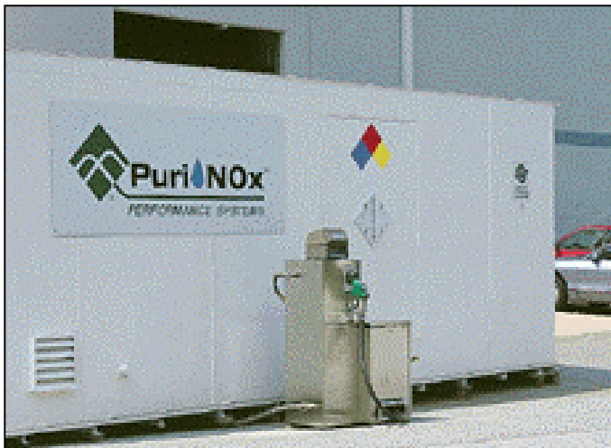
Emulsified Fuel Manufacturing Facility in Dixon, Ca
