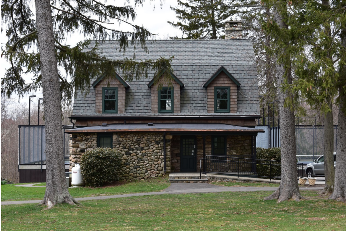
Photo 36. Superintendent's House, looking west.
