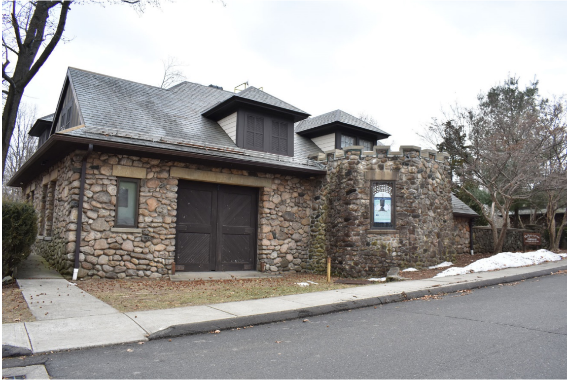
Photo 34. Power House, looking southeast.
