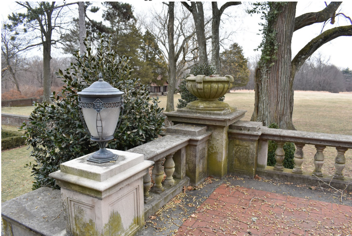
Photo 17. Wavely House terrace balustrade, looking southeast.
