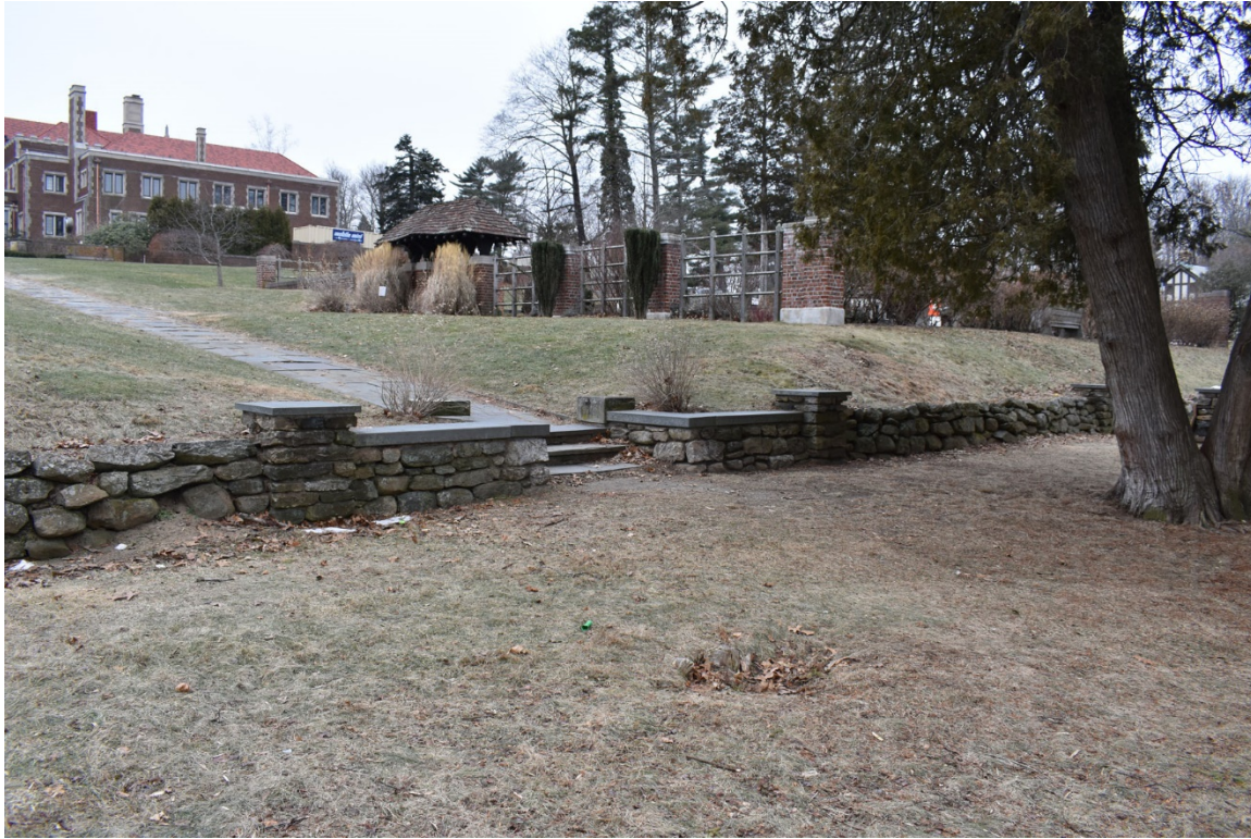
Photo 26. Axial Walk, Rose Garden, Stone retaining wall and steps to east of Waveny House, looking northwest.
