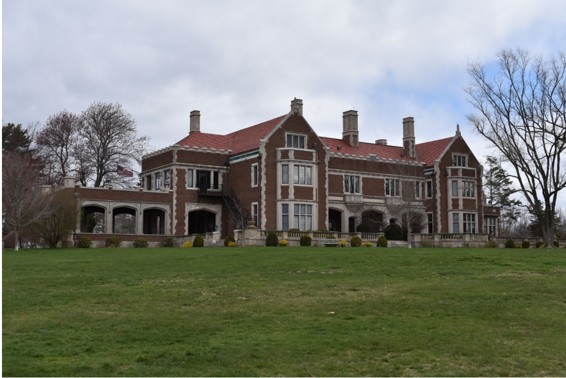
Photo 14. Wavy House, south and west elevations, looking northeast.
