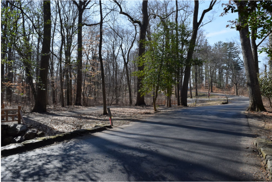
Photo 8. Vehicular Circulation System, Walking Trails Bridges, Stone Bridge, looking west.
