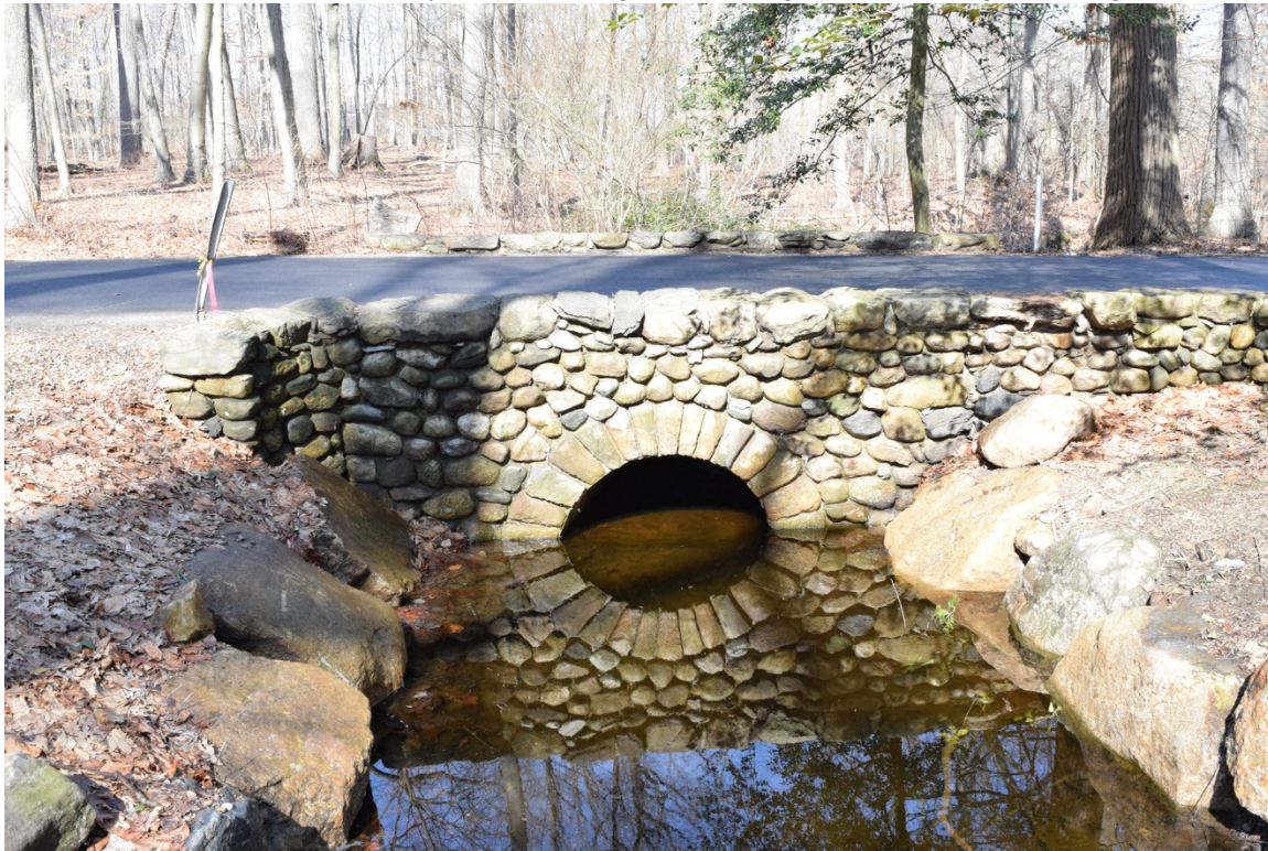
Photo 9. Stone Bridge, looking north.
