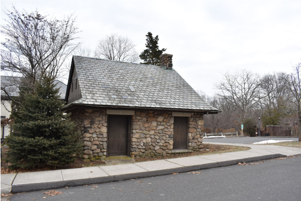
Photo 33. Potting Shed, looking southeast.
