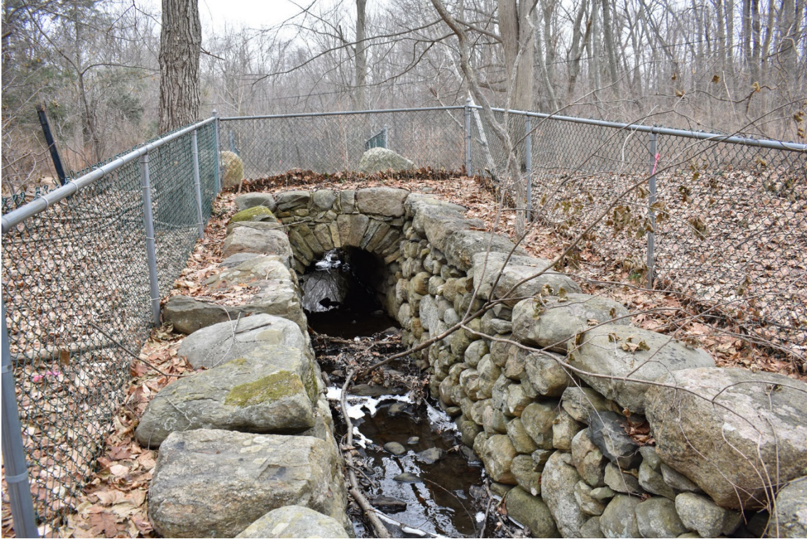
Photo 32. Ice Pond Stone Bridge and Channel, looking north.
