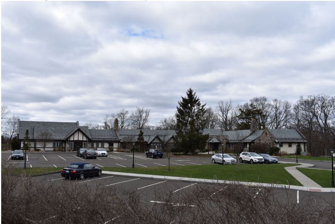
Photo 37. Bungalow, looking southwest.
