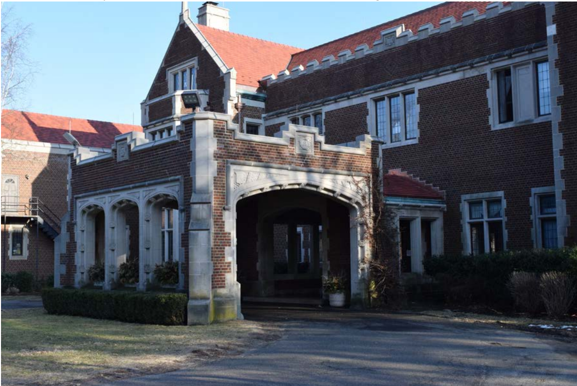
Photo 13. Wavy House Porte-Cochère, looking southeast.
