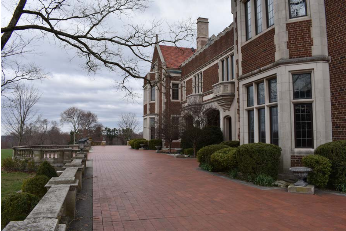
Photo 16. Wavely House terrace and loggia, looking west.
