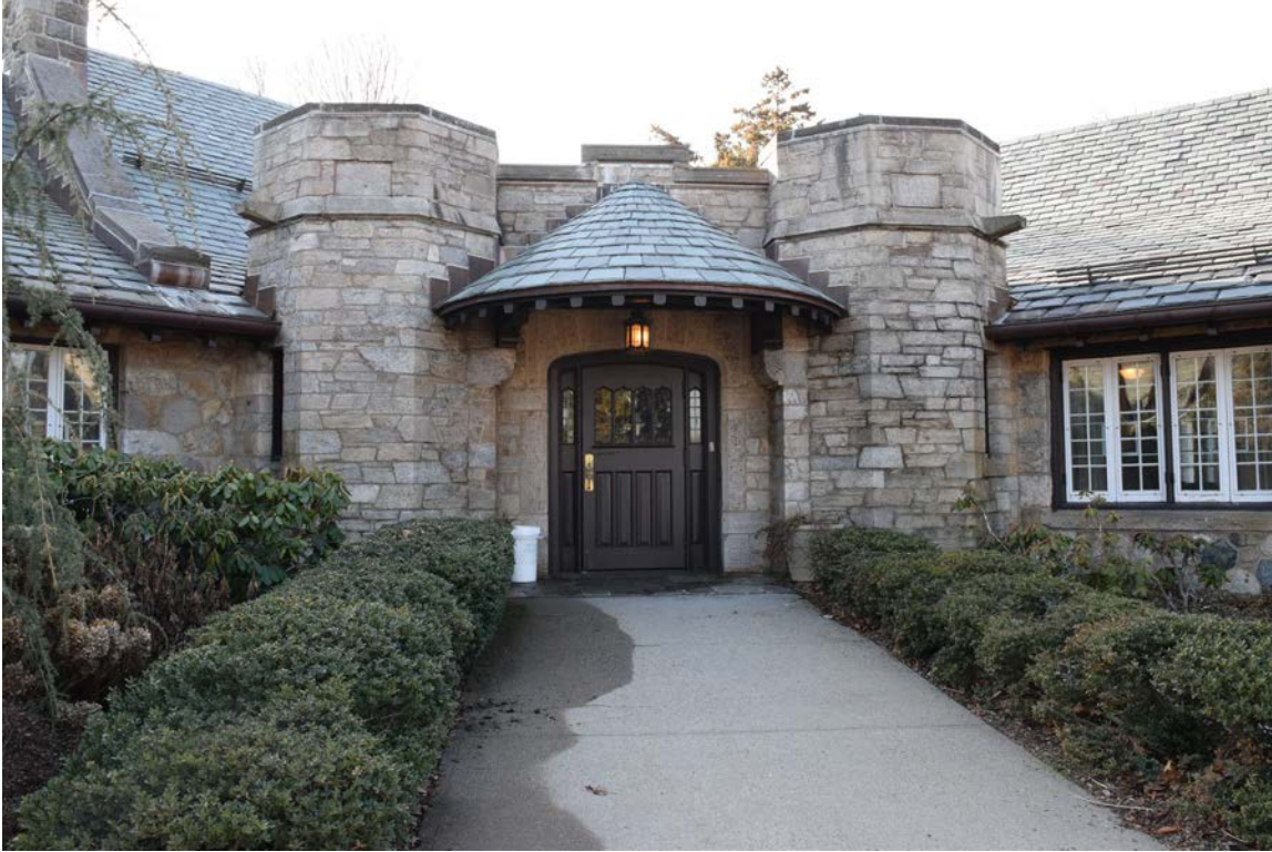
Photo 38. Bungalow entrance, looking west.
