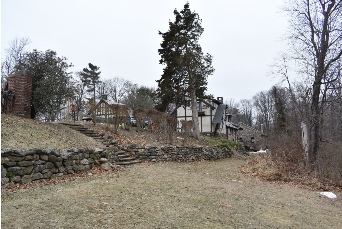
Photo 30. Retaining Wall and Service Cluster , looking northwest.
