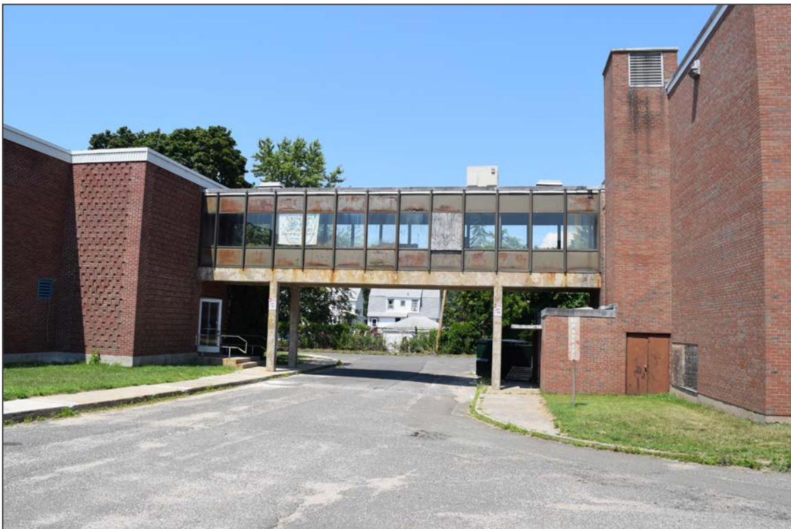
8. Facing southwest toward the west elevation of the bridge connector
