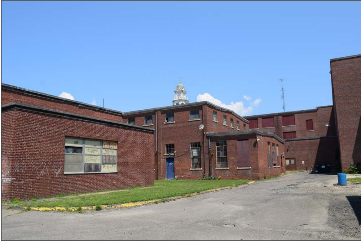
13. Facing northwest toward gymnasium wing addition (left), auditorium (center), south elevation of the 1936 building (right)
