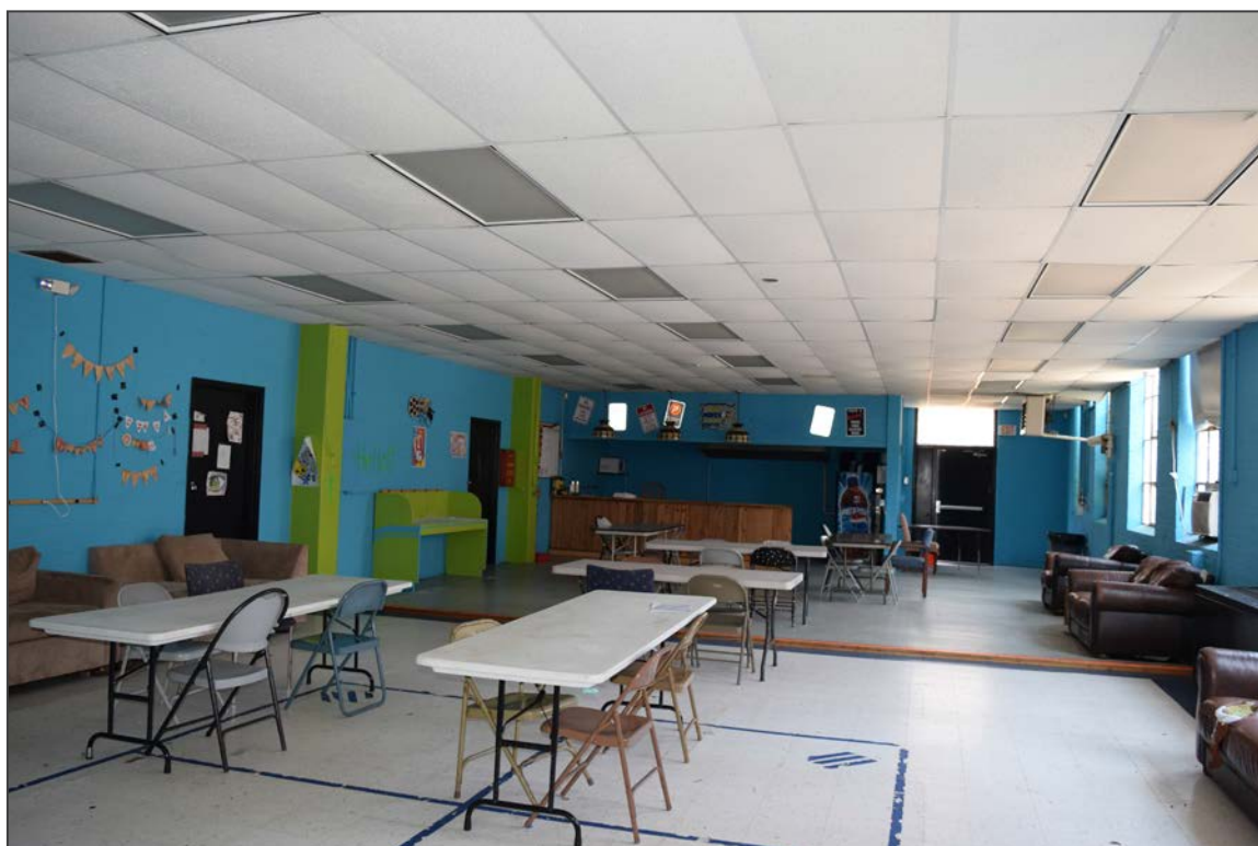
20. Facing west into classroom space of the 1936 Building
