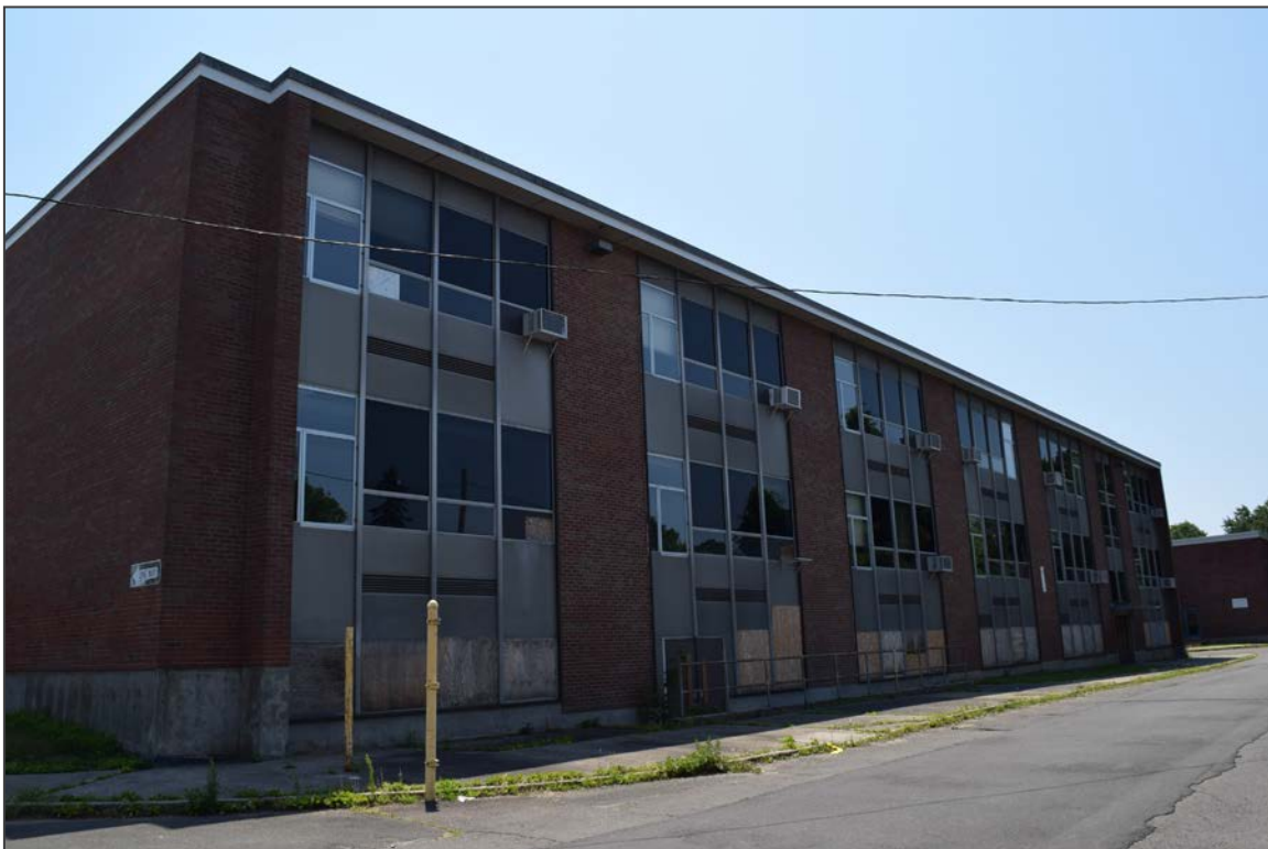
6. Facing southeast toward the west elevation of the 1964 addition
