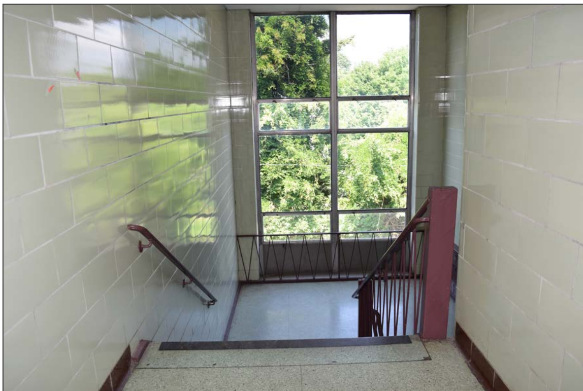
24. Facing east toward second-floor stair in the 1964 addition
