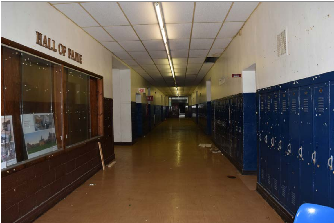
16. Facing west down the first-floor corridor of the 1936 Building
