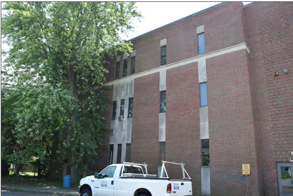
4. Facing southeast toward the north elevation of the 1973 addition
