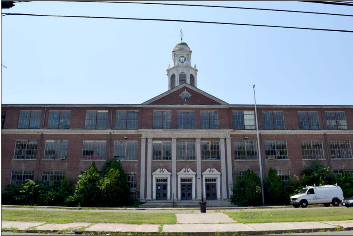
1. Facing south toward the north elevation of the 1936 Building
