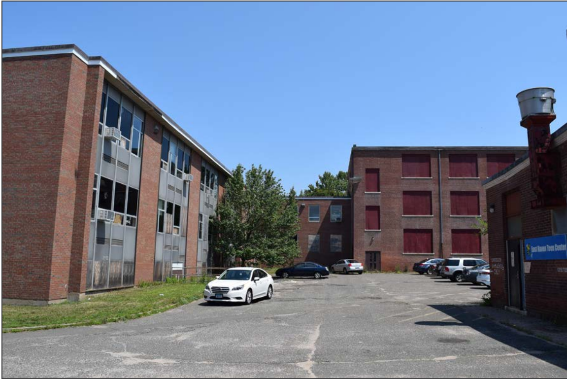
9. Facing north toward the west elevation of the 1964 Building (left) and the south elevation of the 1936 Building
