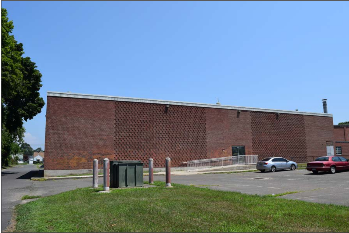
11. Facing northeast toward the south elevation of the pool addition
