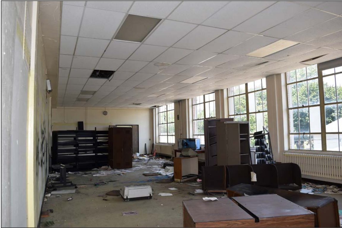
21. Facing northwest into a second-floor classroom of the 1936 Building
