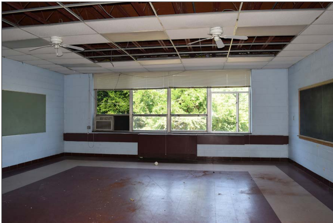
23. Facing west into first-floor classroom space of the 1964 addition
