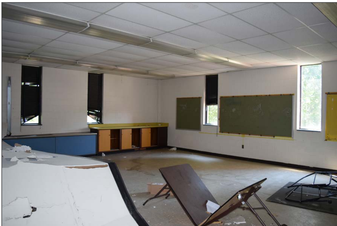
26. Facing southeast into a second-floor classroom of the 1973 addition
