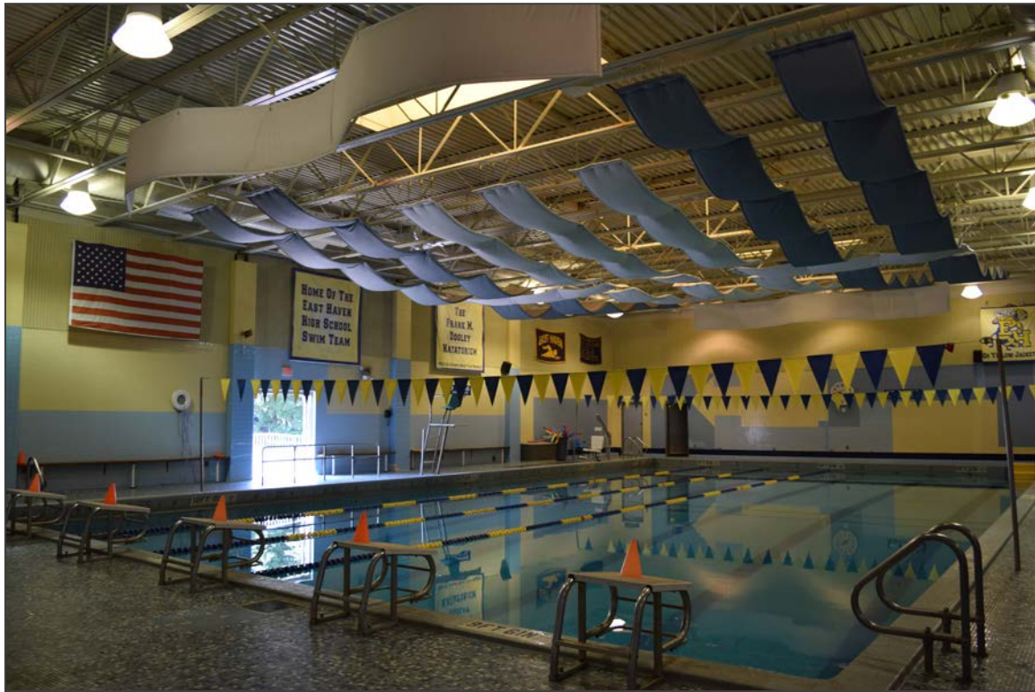
27. Facing southwest toward pool in the 1973 pool addition
