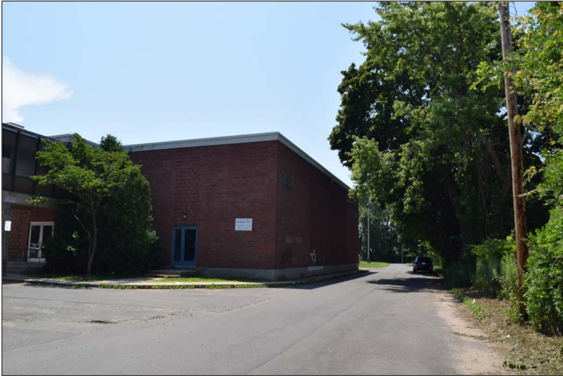
7. Facing southeast toward the north elevation of the pool addition
