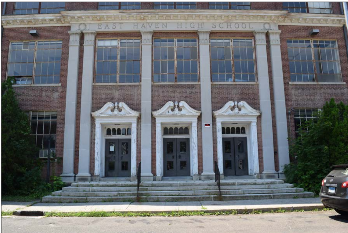
2. Facing south toward the north elevation of the 1936 Building
