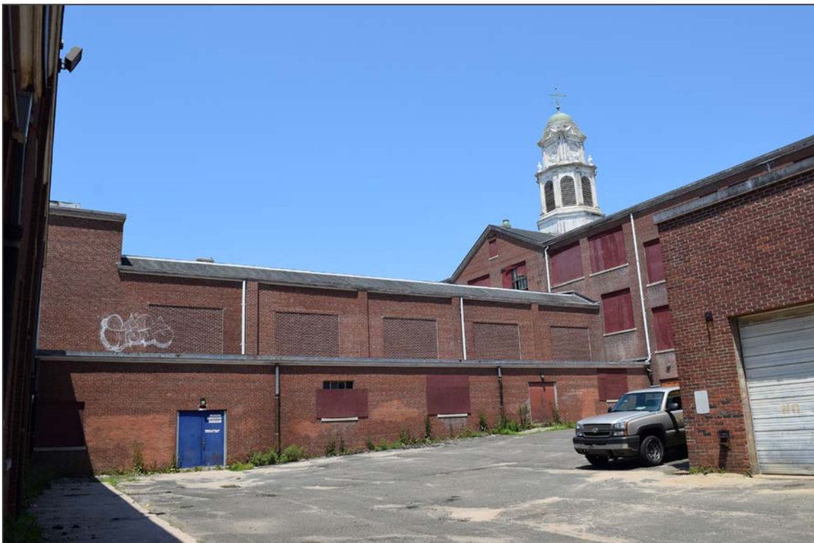
14. Facing northwest toward the east elevation of the auditorium section
