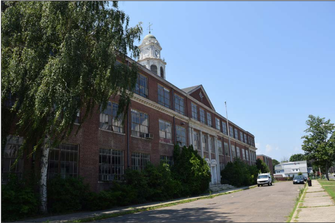
3. Facing southwest toward the north elevation of the 1936 Building
