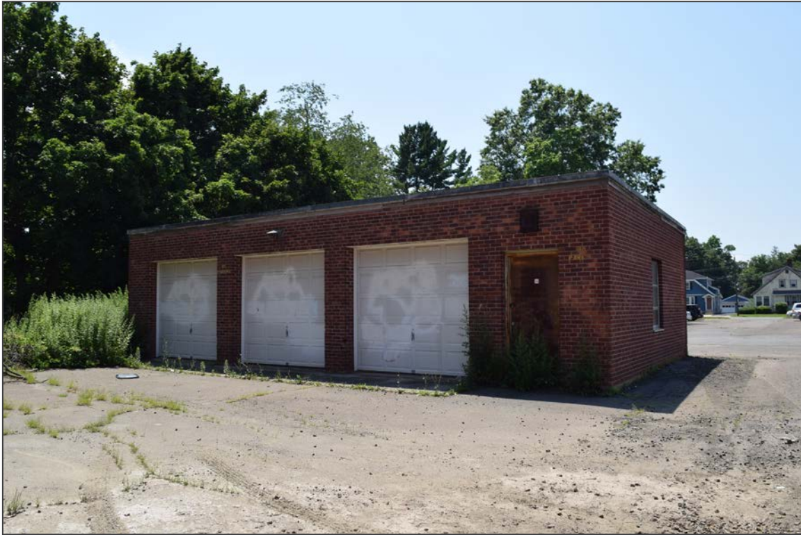
15. Facing southeast toward one-story 1973 garage
