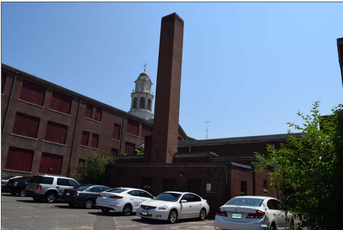
10. Facing northeast toward the south elevation of the pool addition
