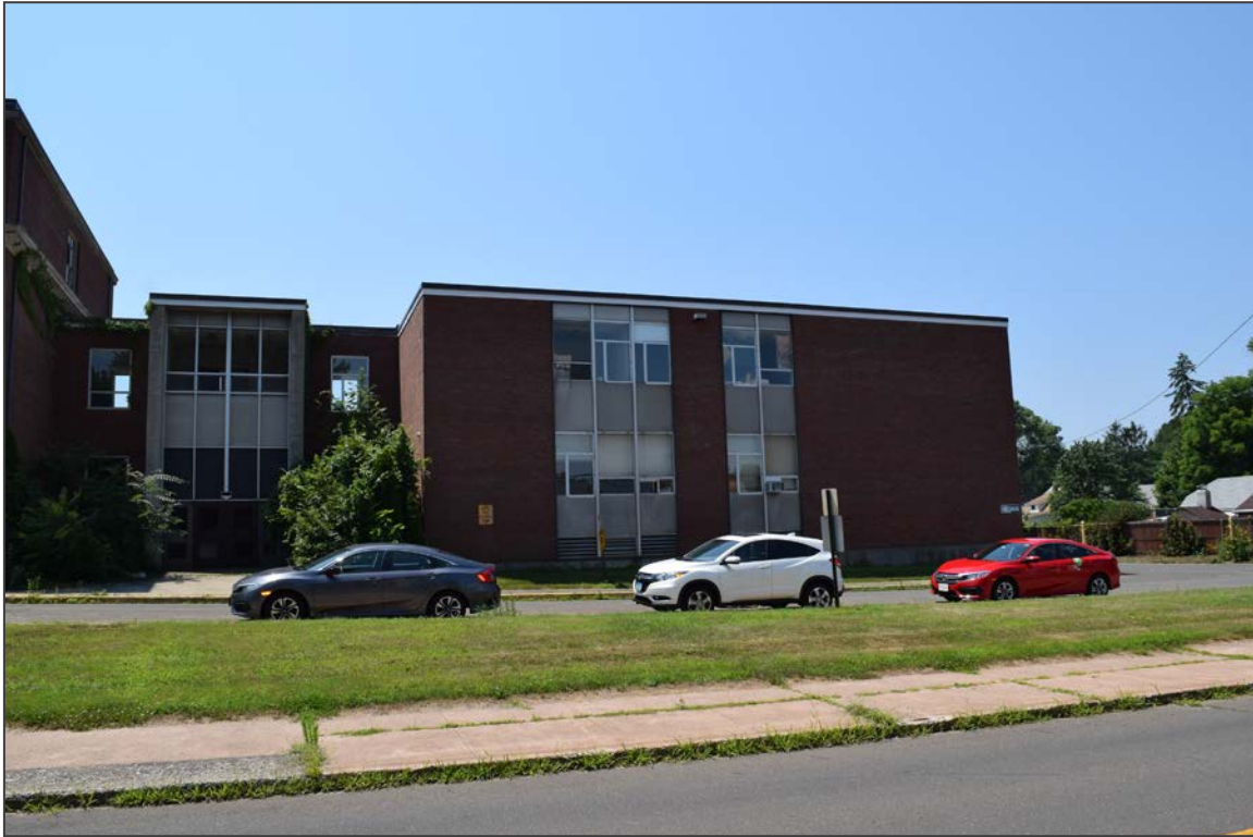
5. Facing south toward the north elevation of the 1964 addition
