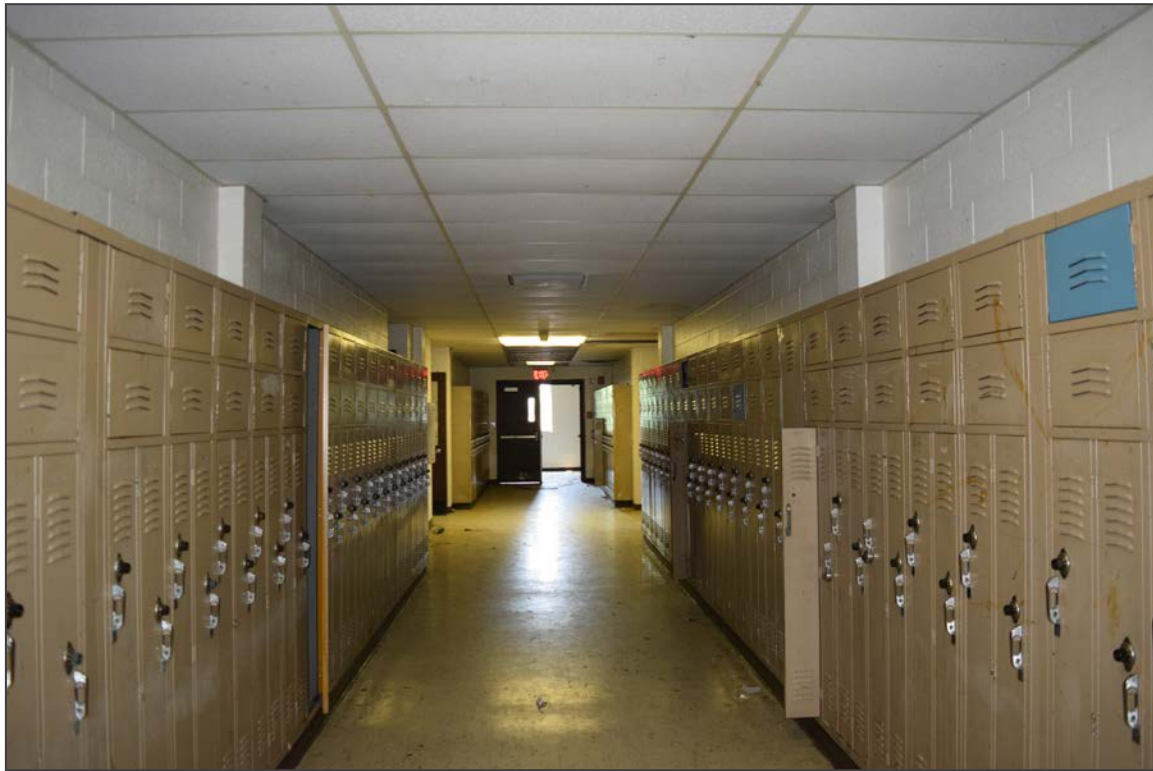
25. Facing south down the second-floor corridor of the 1973 addition
