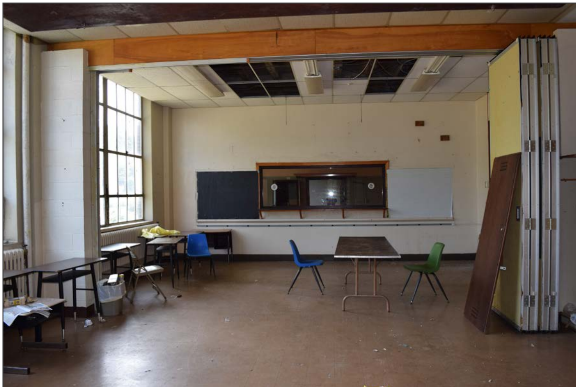
17. Facing east in a first-floor classroom of the 1936 Building
