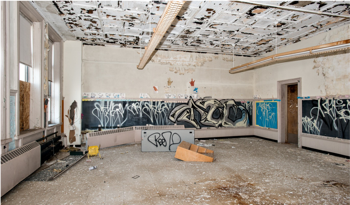
Photo 15. Interior view west showing original paneling, moldings, plaster walls, flooring, stamped metal ceiling and blackboards in typical classroom on north side of elementary school.
