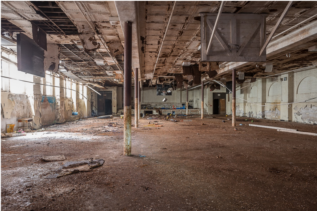
Photo 22. Interior view east showing gymnasium with niches on south wall.
