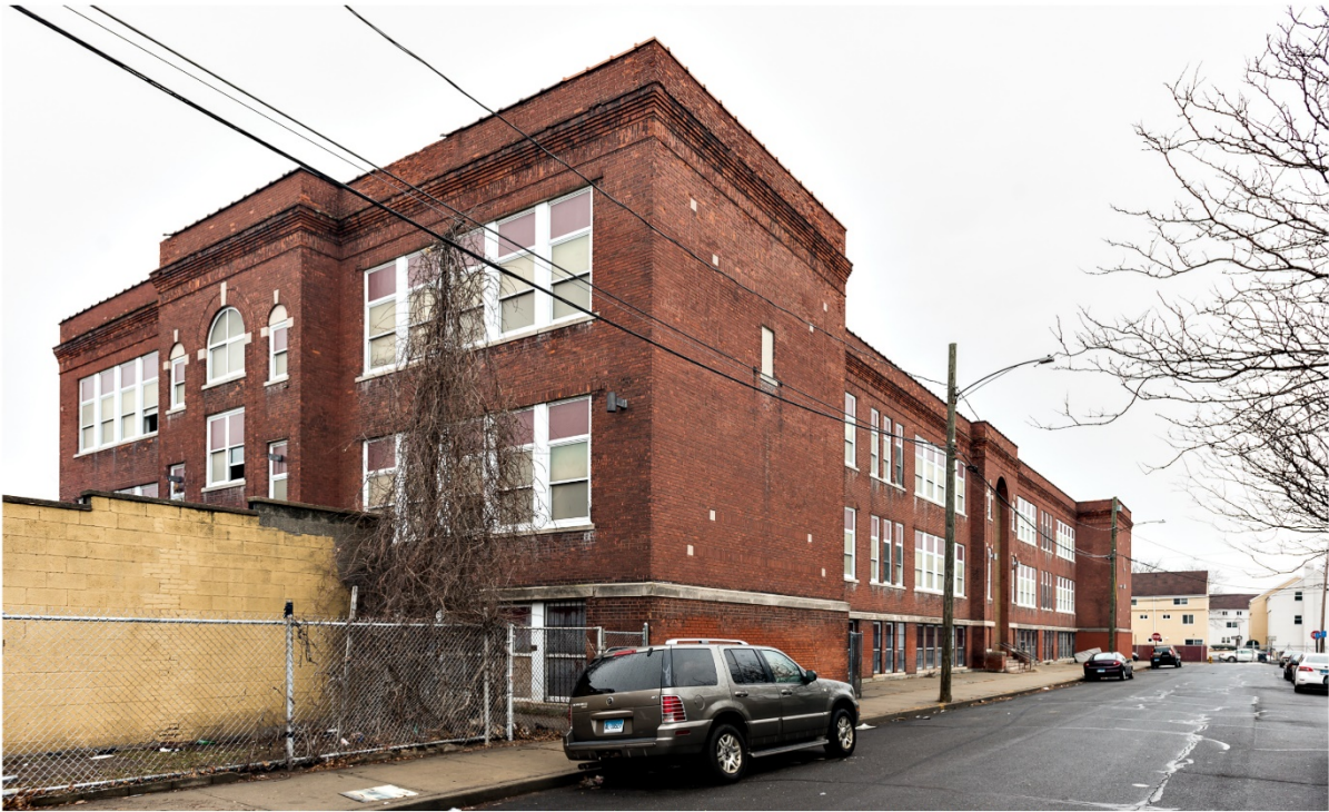
Photo 9. View northeast showing west elevation and facade of junior high school.
