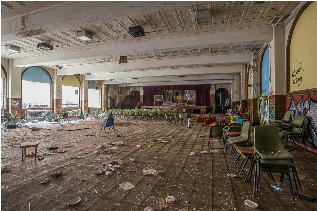
Photo 24. Interior view east showing auditorium of junior high school.
