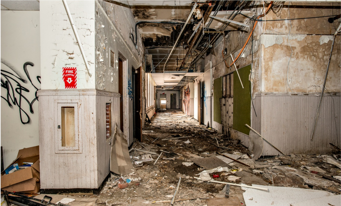
Photo 16. Interior view east showing second floor corridor of elementary school.
