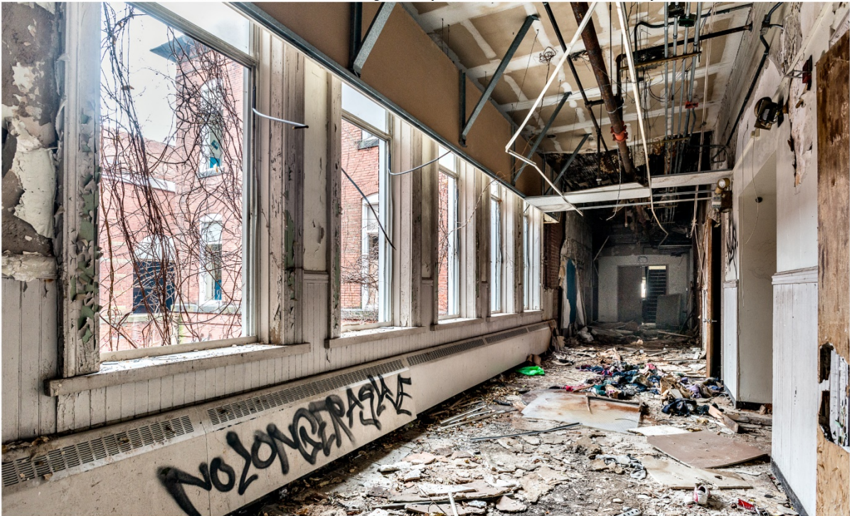
Photo 12. Interior view southwest showing first floor corridor of elementary school.
