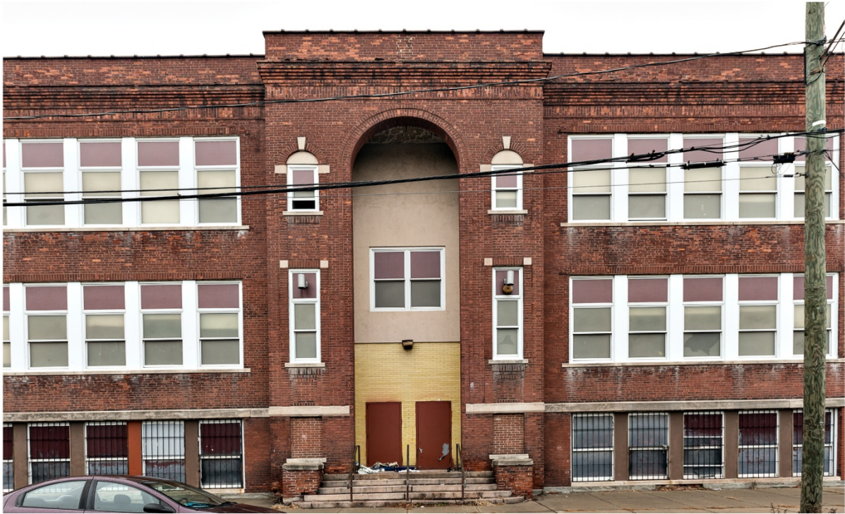
Photo 7. View north showing center entrance on facade of junior high school.
