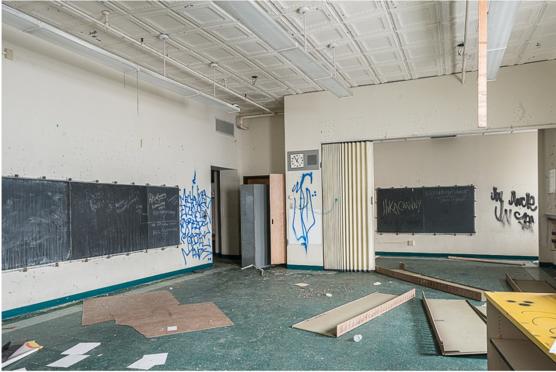
Photo 27. Interior view southeast of typical junior high school classroom.
