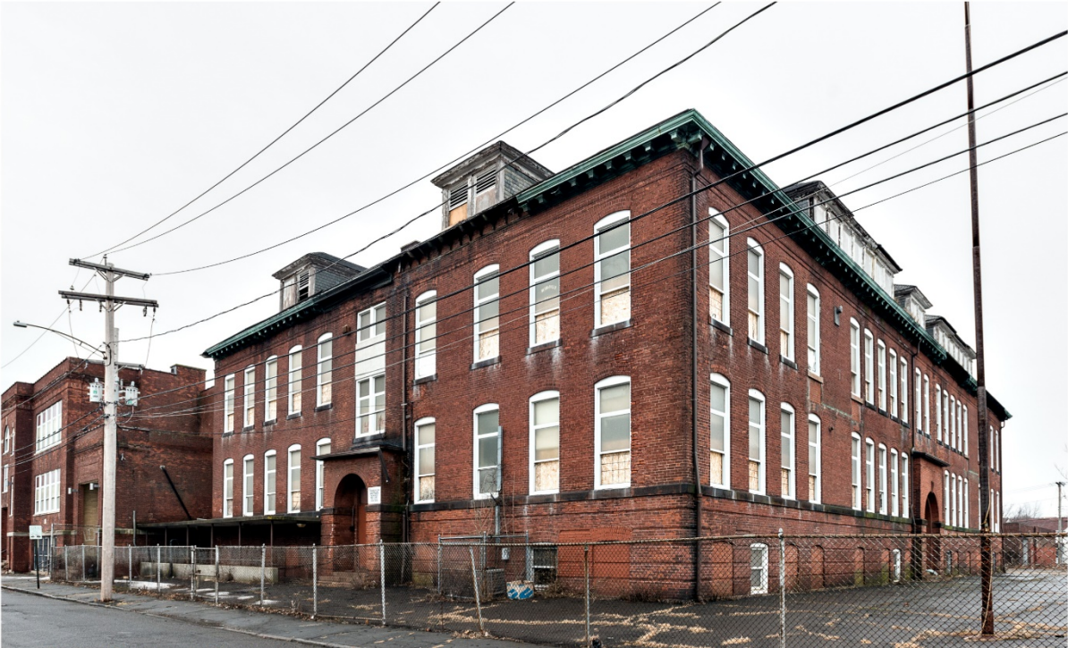
Photo 1 Waltersville School. View southwest showing facades on Gilmore Street and north elevation of elementary school.
