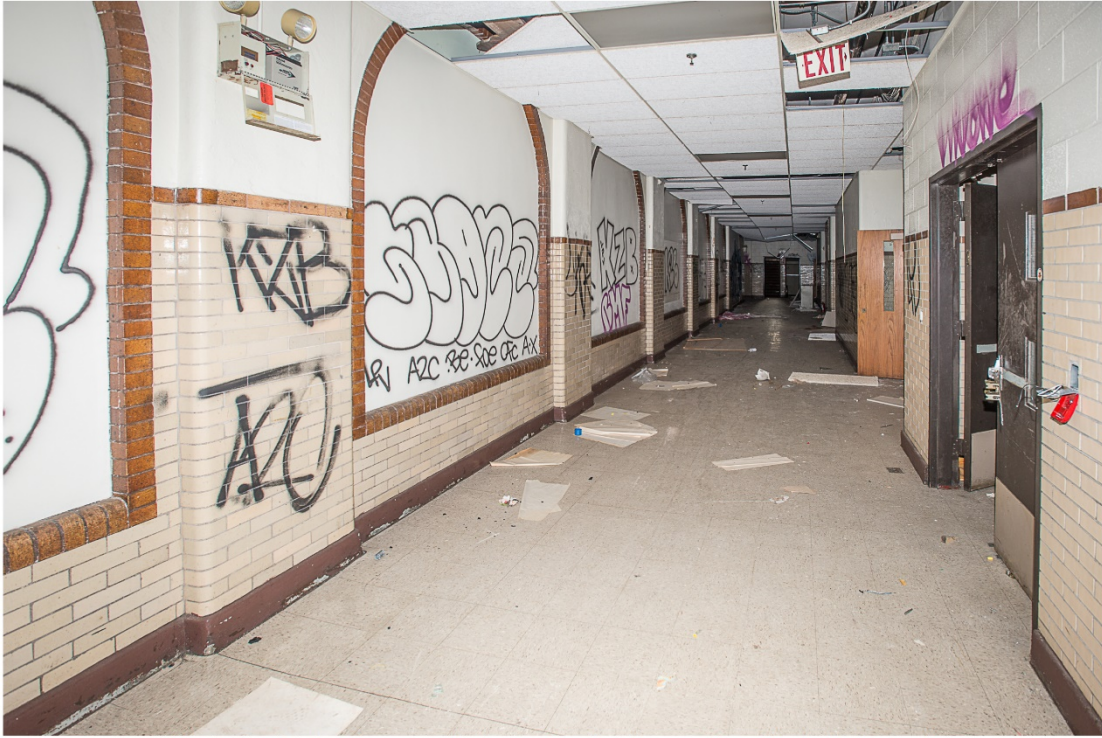
Photo 23. Interior view east showing corridor first floor corridor of junior high school.
