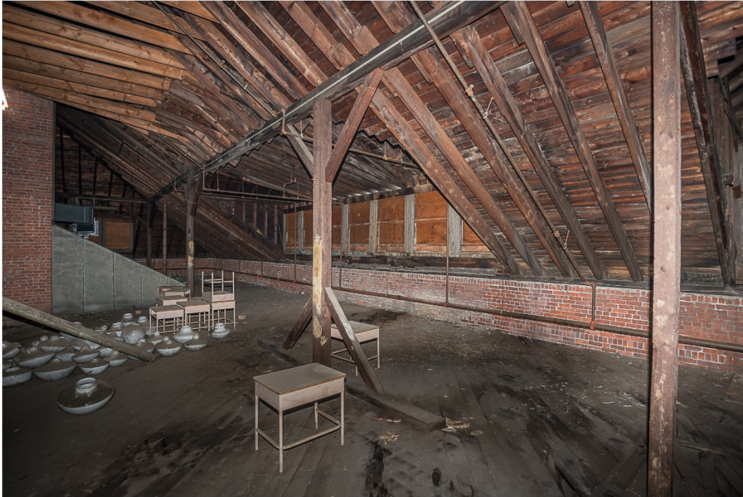
Photo 19. Interior view northwest showing wood floor, brick knee walls, dormers and exposed wood structure in attic of elementary school.
