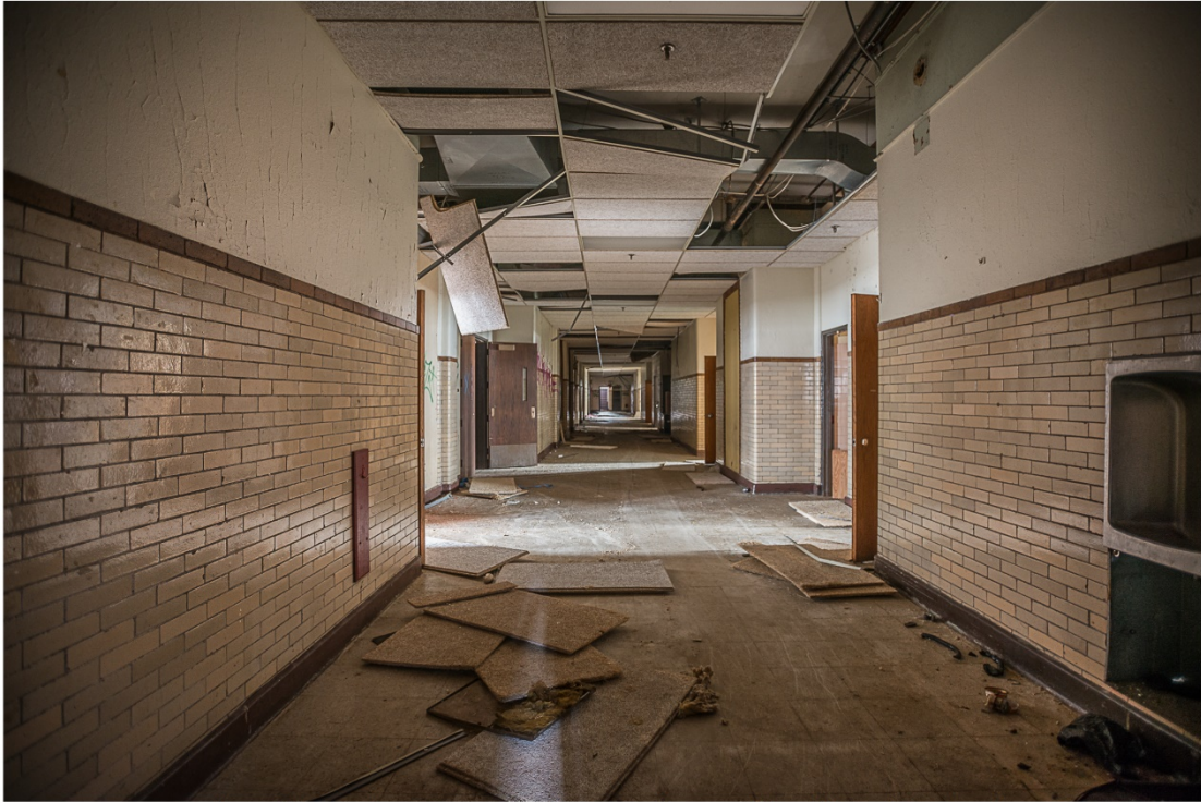
Photo 25. Interior view east showing second floor corridor of junior high school.
