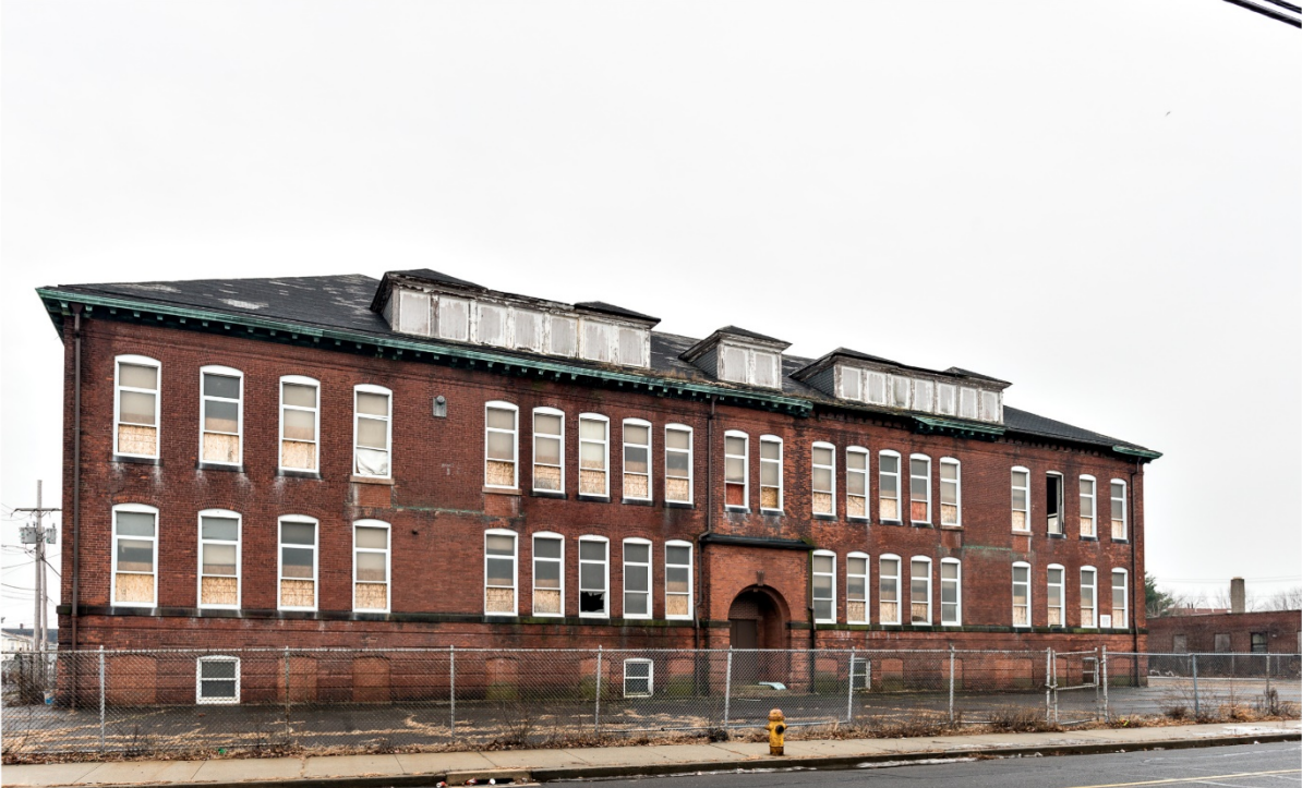
Photo 2. View south showing north elevation of elementary school.
