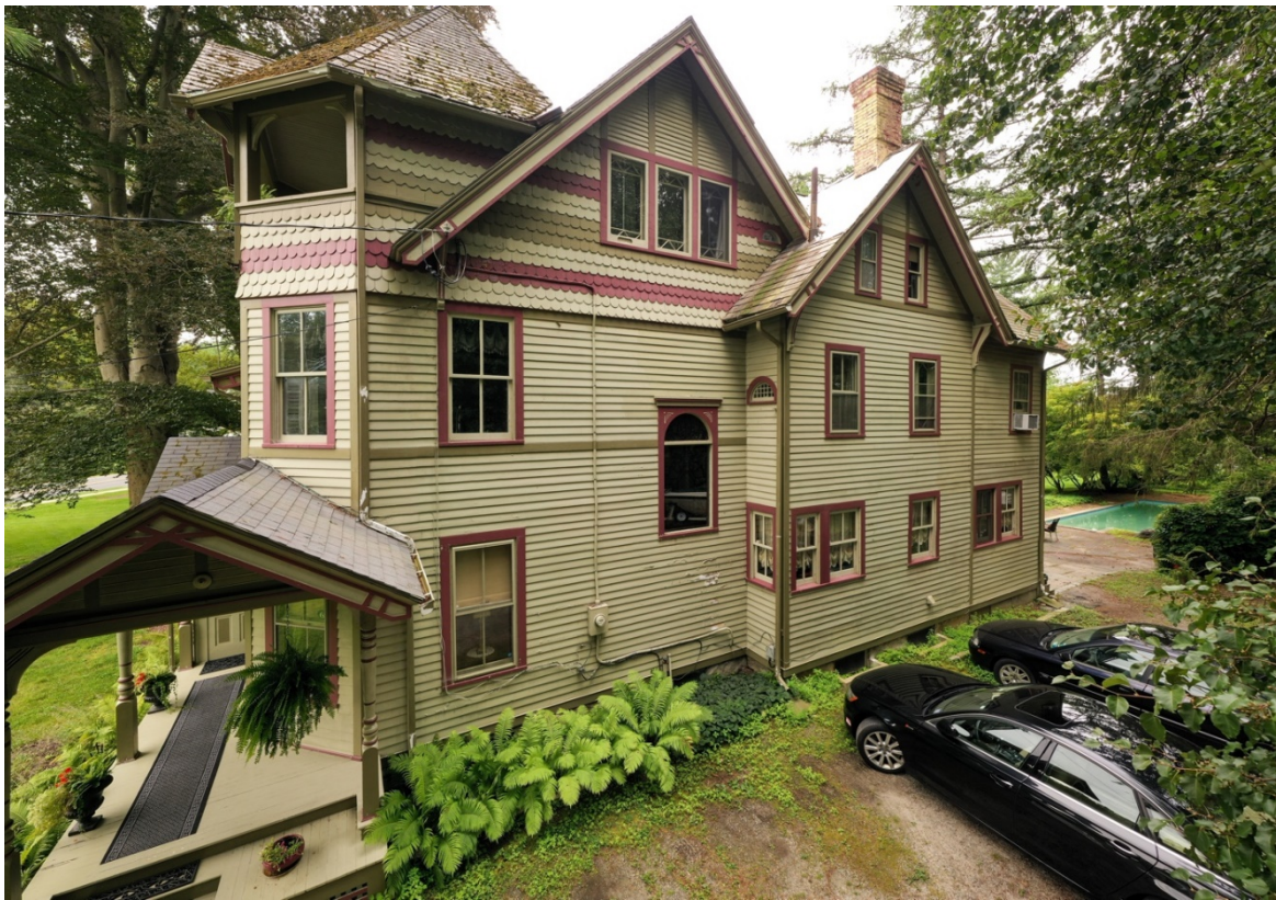
Photo 4 of 23: Northeast elevation, camera facing southwest.
