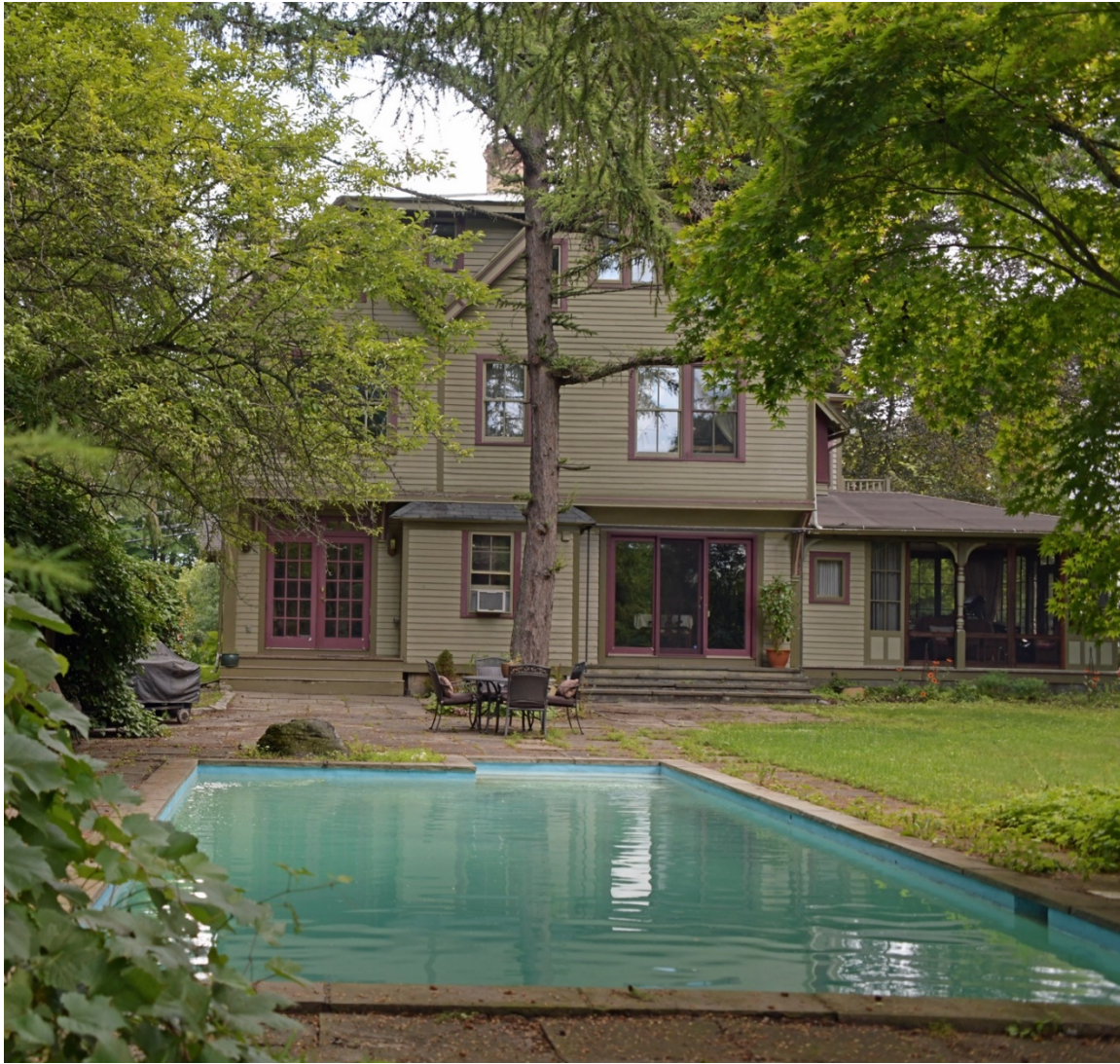
Photo 15 of 23: West elevation and in-ground pool, camera facing east.
