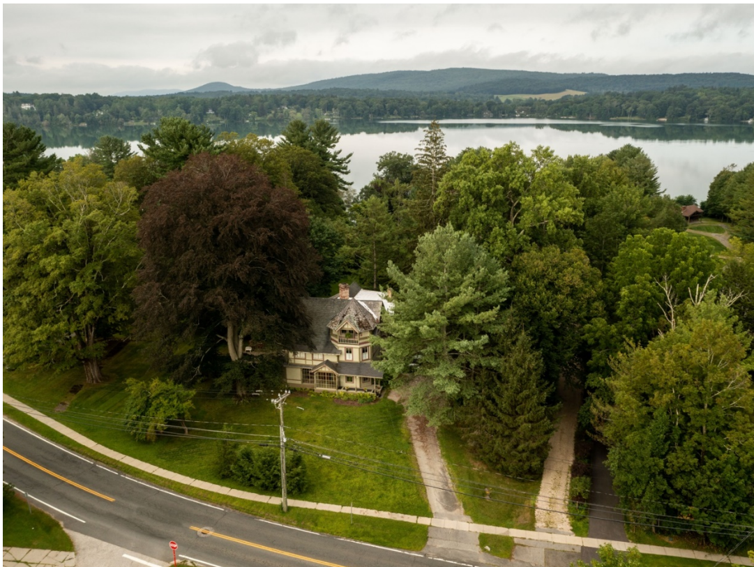
Photo 2 of 23: Aerial view of east façade, camera facing west.
