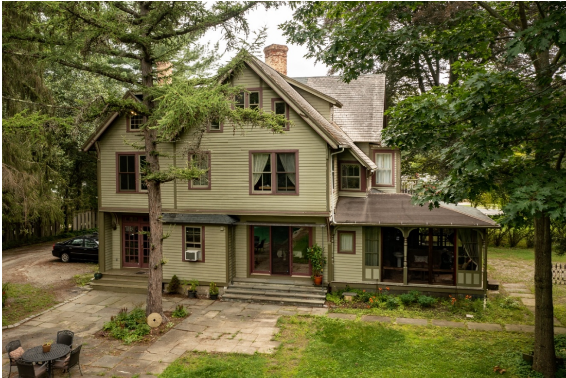
Photo 3 of 23: West elevation, camera facing east.
