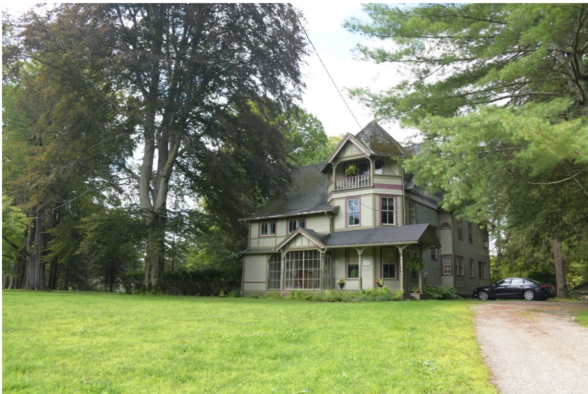
Photo 6 of 23: East façade, camera facing west.
