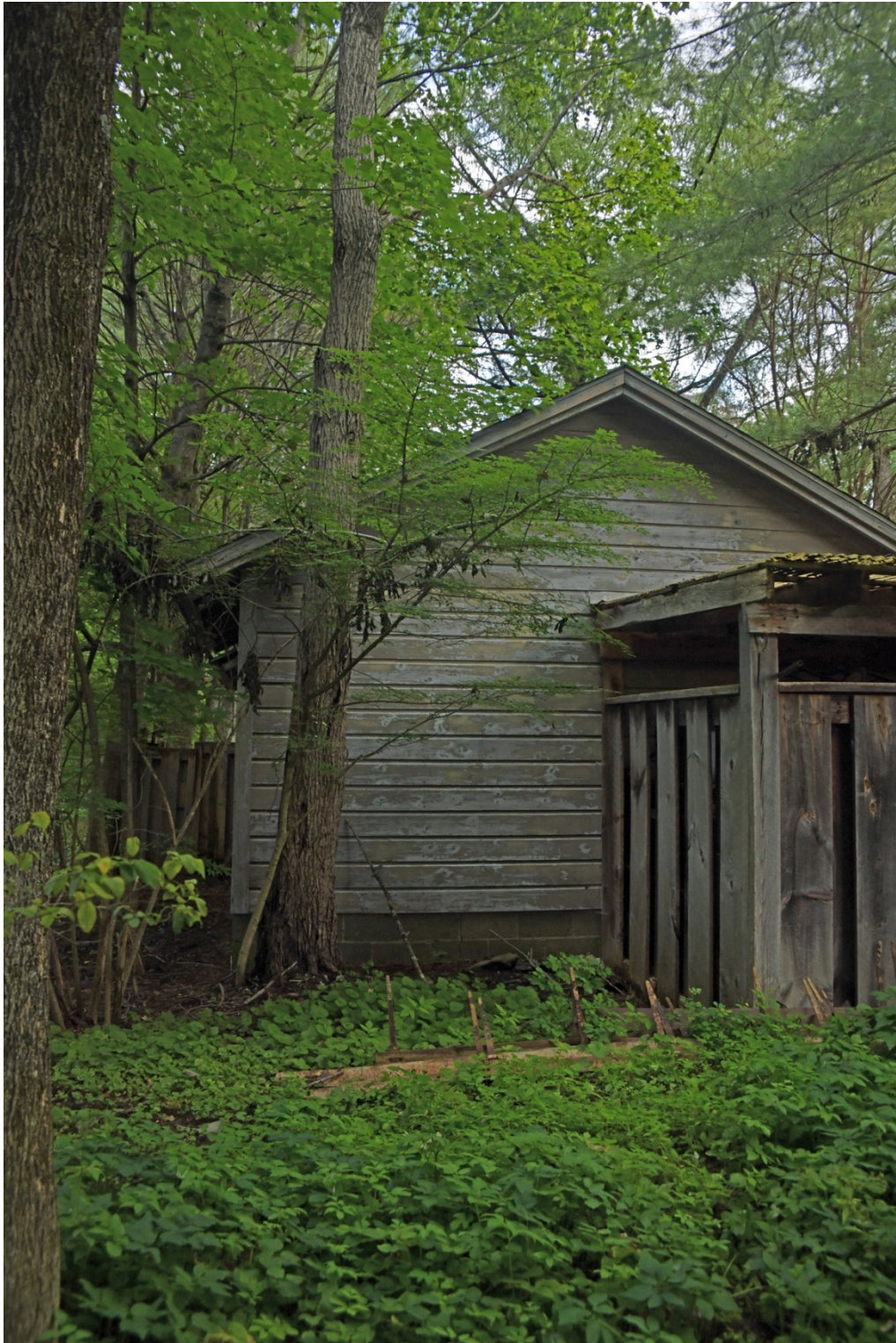
Photo 17 of 23: West elevation of garage, camera facing east.
