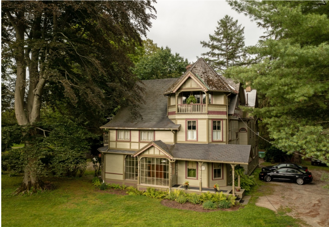
Photo 1 of 23: East façade, camera facing west.
