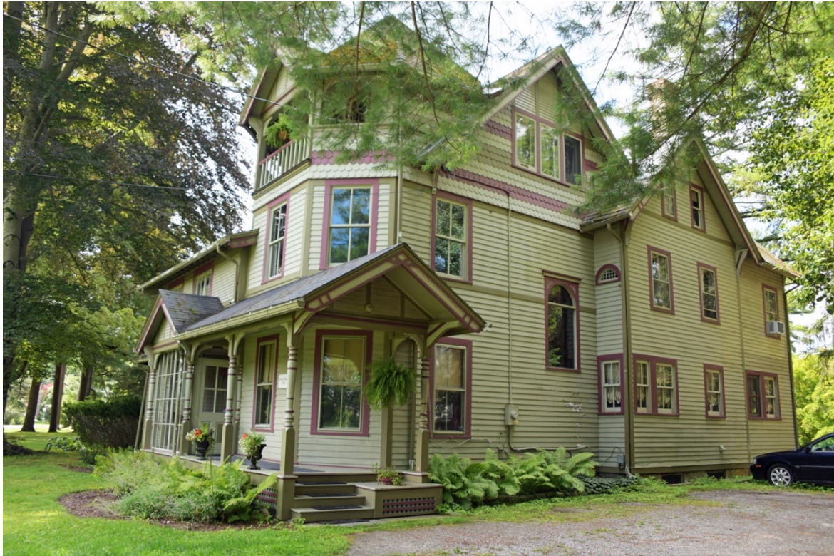
Photo 12 of 23: Northeast elevation, camera facing southwest.
