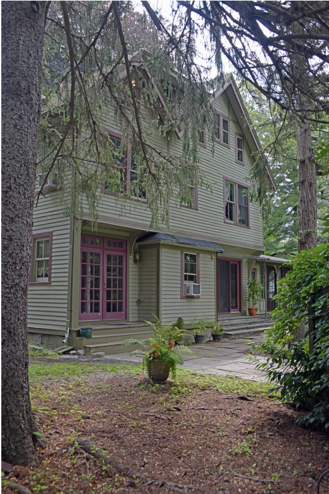
Photo 14 of 23: Northwest elevation, camera facing southeast
