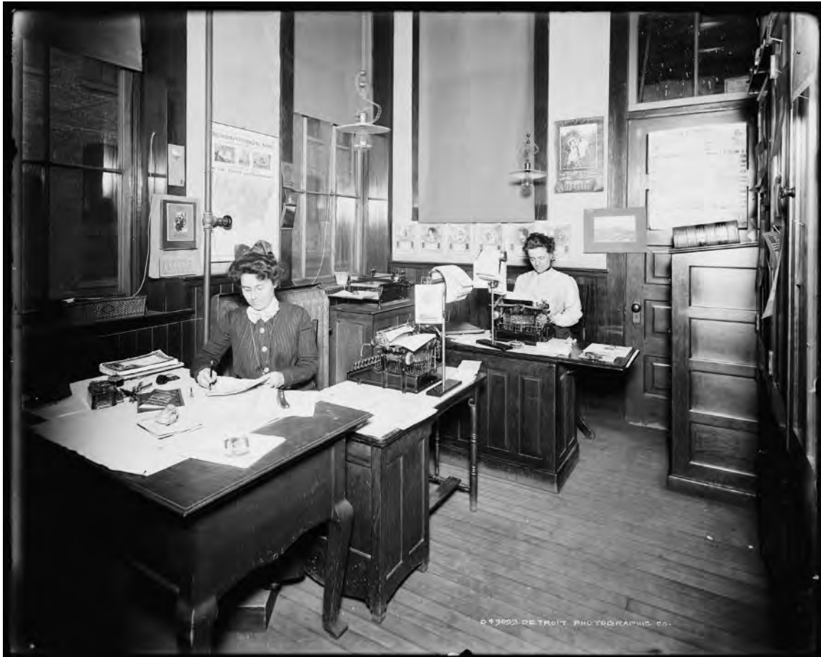
Stenographers' room, Leland & Faulconer Manufacturing Co., Detroit, MI, 1903 (LOC P&P, Detroit)
