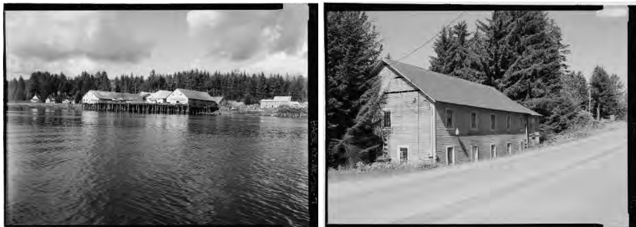
(L) Kake Cannery, Alaska, manager's houses on left, 2000 (Jet Lowe, LOC P&P, HAER AK-26) (R) Kake Cannery, bunk house for white workers, 2000 (Jet Lowe, LOC P&P, HAER AK-26)
