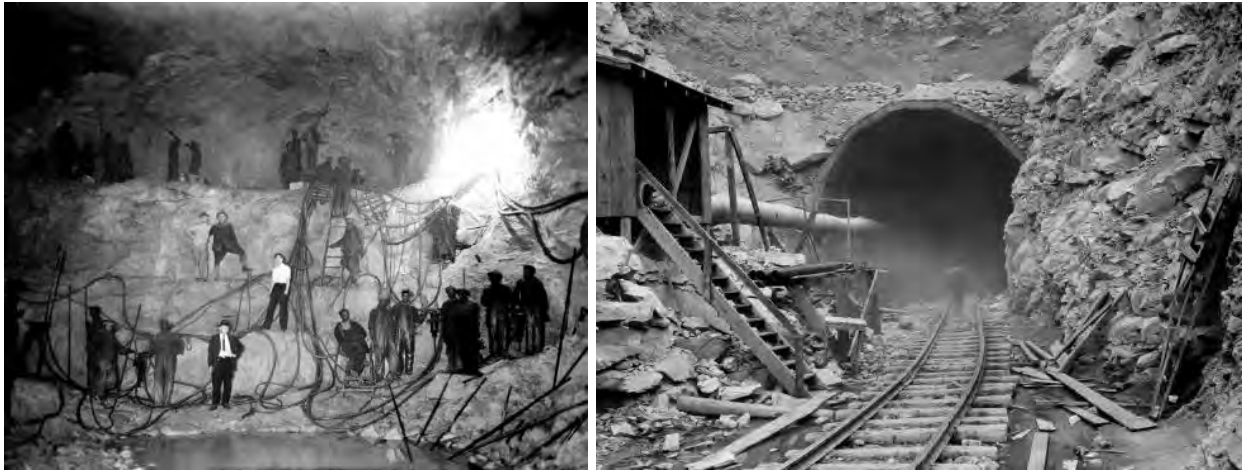
To create the Hawks Nest Tunnel, workers had to drill through nearly pure sandstone, which produced clouds of toxic silica dust. Workers in these photos are not wearing respirators — a requirement mandated by Congress after hundreds of men died from exposure to silica in the tunnel; (L) Drilling crew posing in tunnel; (R) Worker emerging from dust-filled tunnel, Hawks Nest Tunnel, Hawks Nest-Gauley Junction, WV, 1931 (West Virginia State Archives, Elkin Metals Collection)
