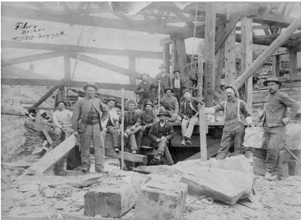
Construction crew on the Delaware, Lackawanna and Western’s Winton Branch, Jessup, MD, 1888 (Steamtown National Historical Park)
