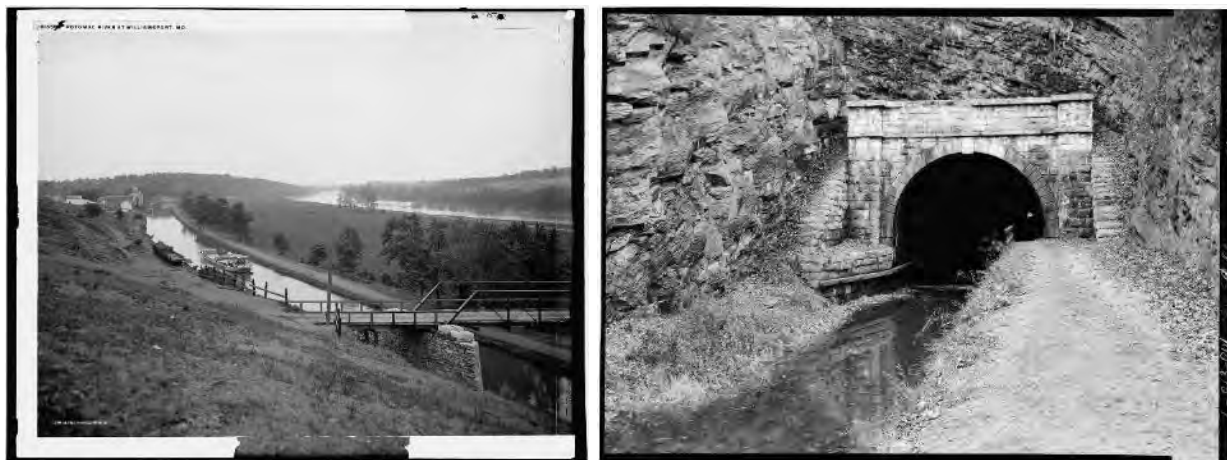
(L) C & O Canal, Williamsport, MD, 1904 (LOC P&P, Detroit) (R) Chesapeake & Ohio Canal, Paw-Paw Tunnel, Allegany County, MD, 1960 (Jack E. Boucher, LOC P&P HABS MD-810))
