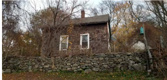
Local Cape Verdeans often collected stones from local farms to build walls like this one, built by Poncho Rodrigues for Joseph C. Delgado, 165 (R) Talman Street.
