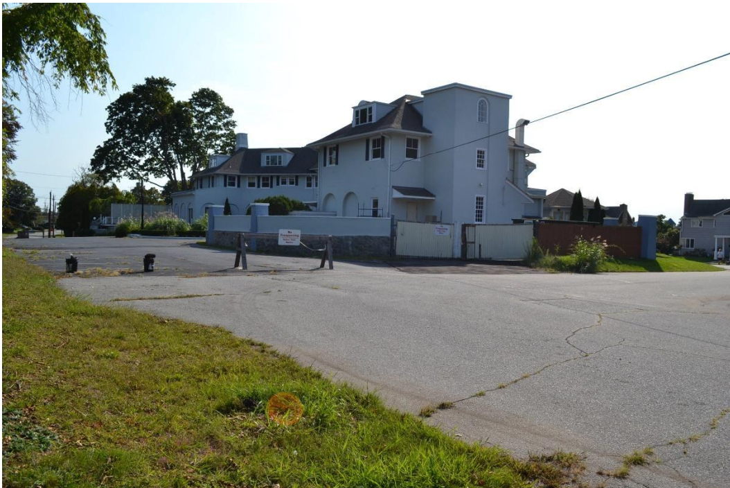
View northeast along Admiral Drive toward the entry court behind the house.
