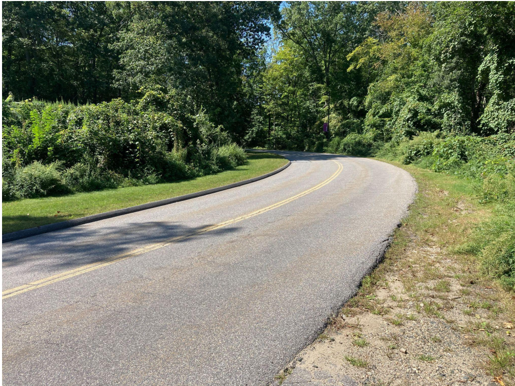
View east along approach road.
