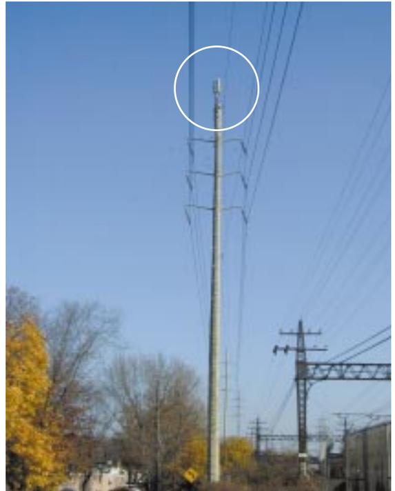
Co-location on an electric transmission structure located on 3 Mechanic Street in Darien.
