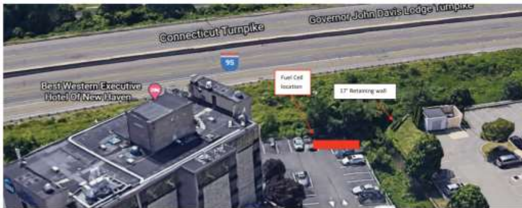
East View of Fuel Cell Site
