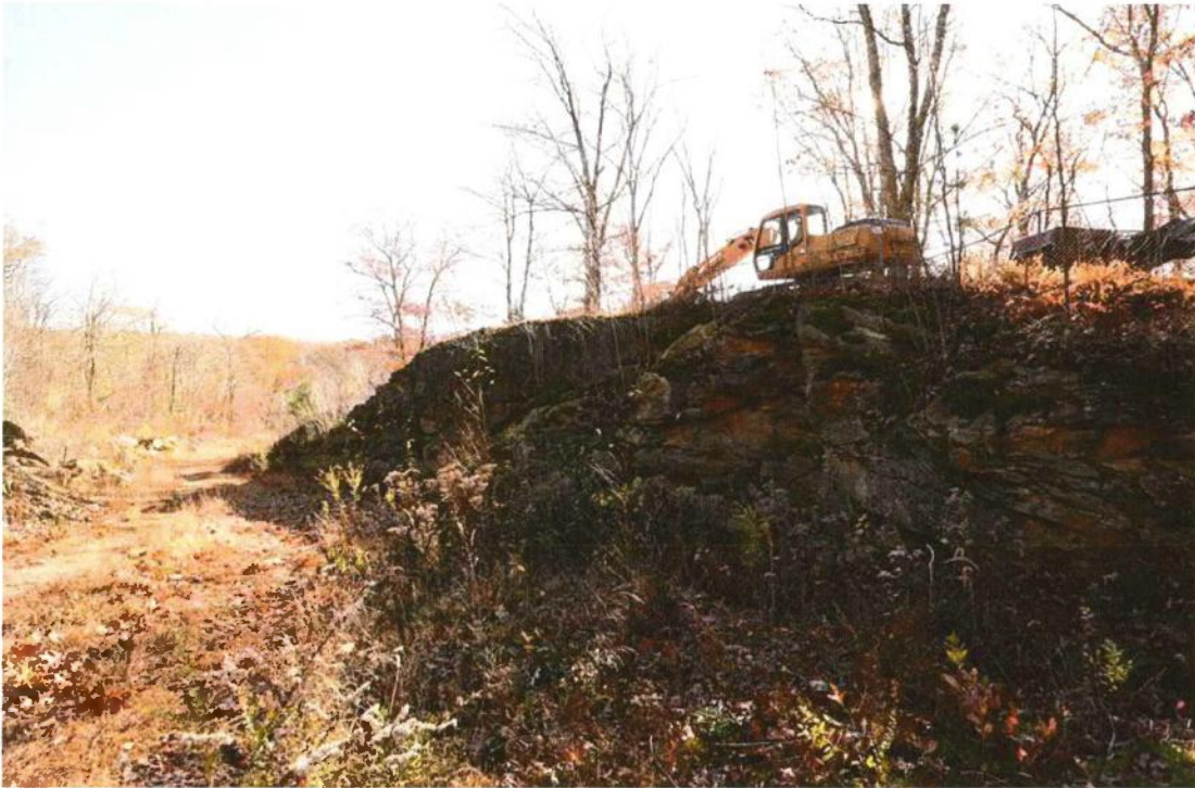
Photo 3: Access road, photo looking east toward Skinner St out of subject property, showing rock cut on the south side of access road exposed during previous construction activities.
