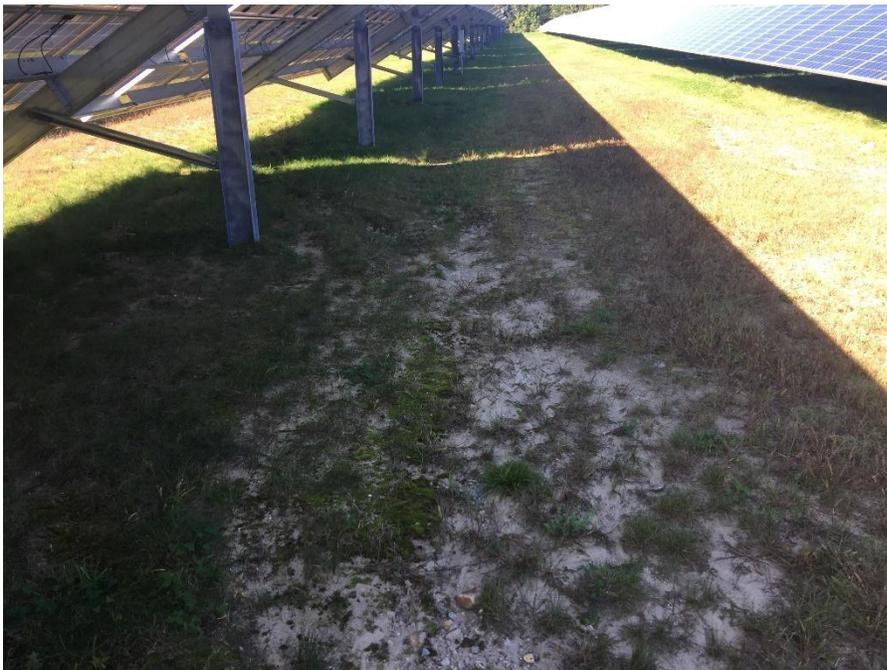
Figure 2 - Erosion & Sedimentation resulting from concentrated flow
