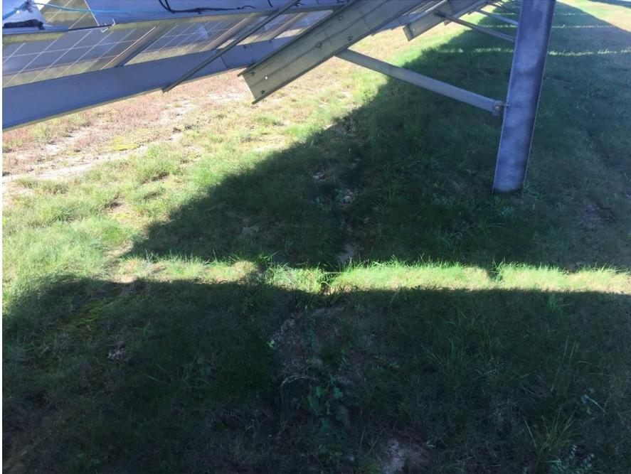
Figure 1 - Concentrated flow from runoff off solar panel
