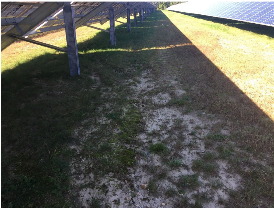
Figure 2 - Sedimentation of eroded material within area of array (East Lyme)
