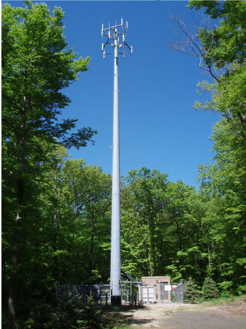
View of Tower and Compound
