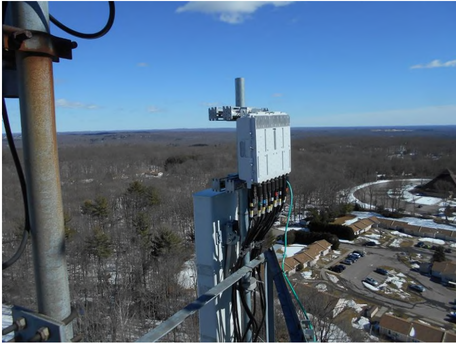
Photos of Sprint's typical existing equipment and mounts at 180'.
