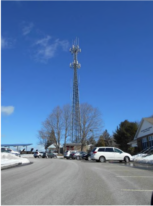
Overview photos of the 190' self-supporting tower located in Coventry, Connecticut.
