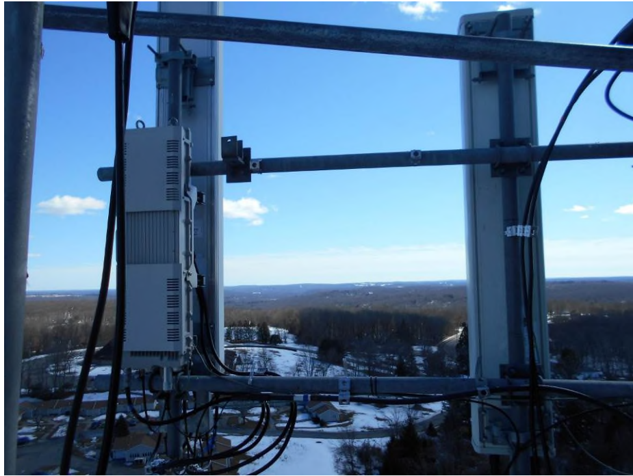
Additional photos of Verizon Wireless's typical existing equipment and mounts at 150'.
