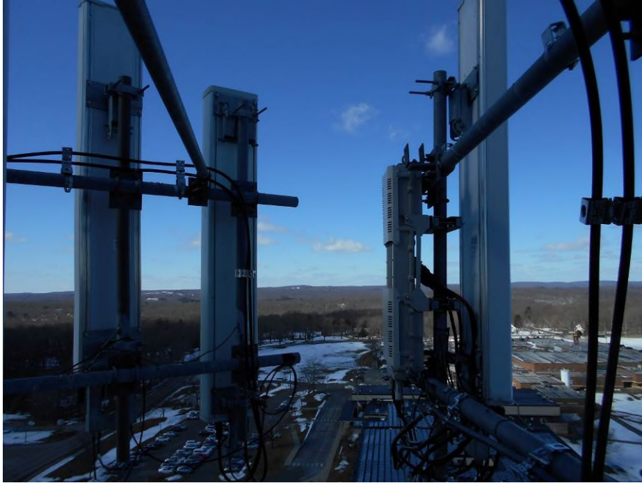
Photos of Verizon Wireless's typical existing equipment and mounts at 150'.
