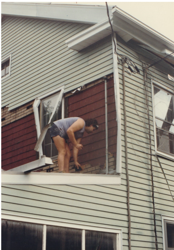
92 Pequot Avenue – Photos provided by the current owner show removal of the exterior cladding ca. 1985.
