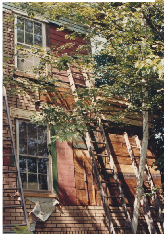
92 Pequot Avenue – Photos provided by the current owner show removal of the exterior cladding ca. 1985.
