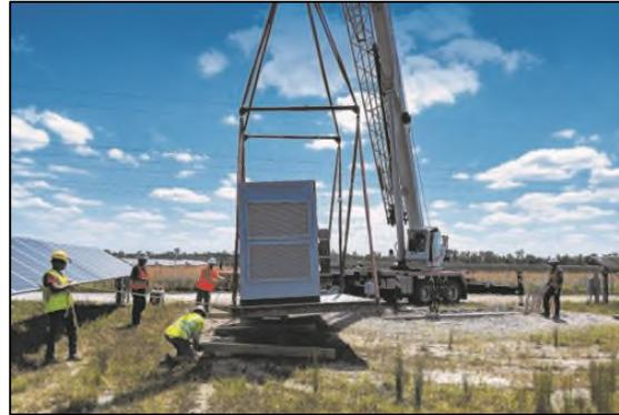
*The process of inverter removal from the site after cable disconnection*
