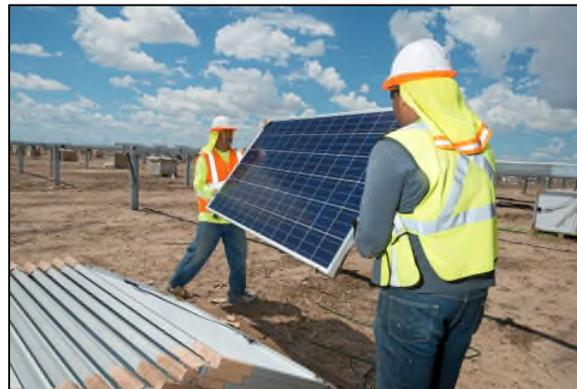
*The process of PV module removal from a rack mounting system*
