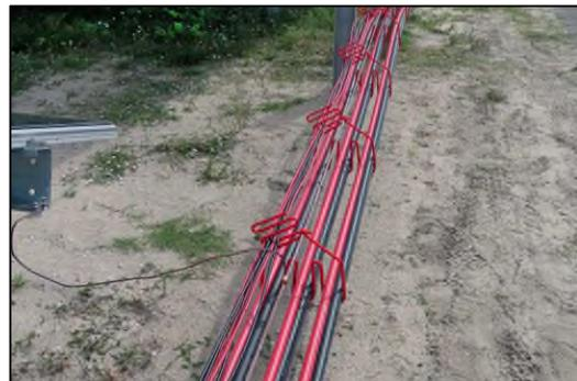
*AC power cable removed from the trench*
