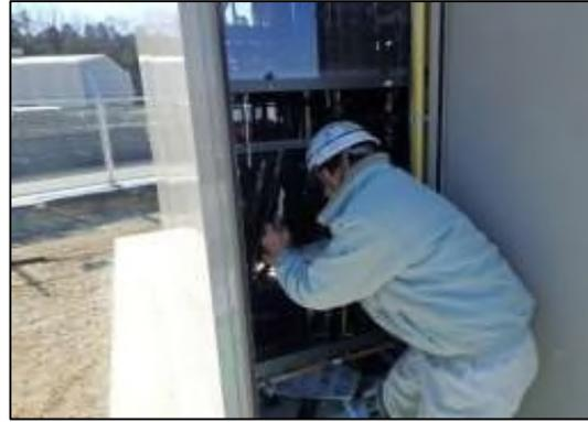
*Power cable disconnection at Solar inverter*
