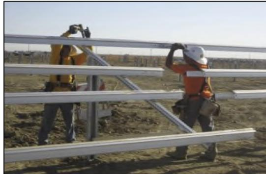
*The process of removing the rack mounting system*
