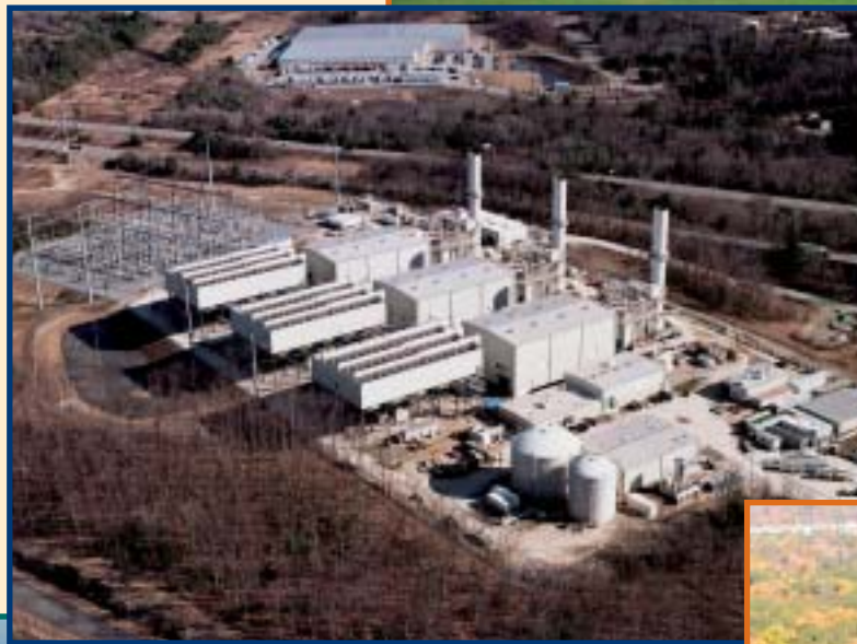
792 MW natural gas-fired electric generating facility, Killingly
