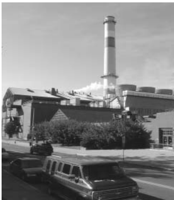
A cogeneration facility in a city setting.
