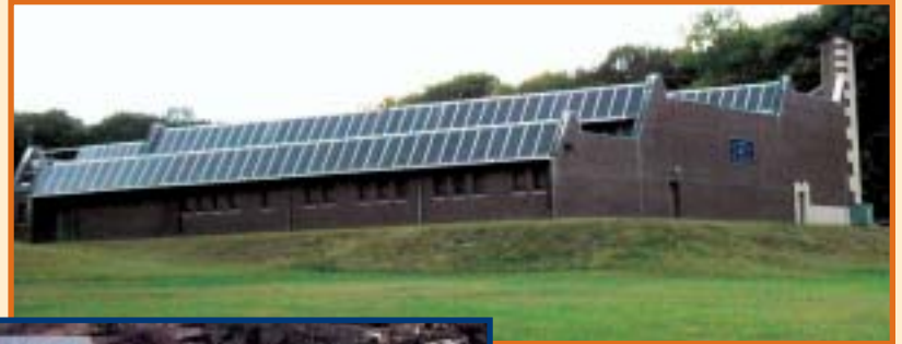
Solar collectors at Connecticut National Guard Center, Norwich
