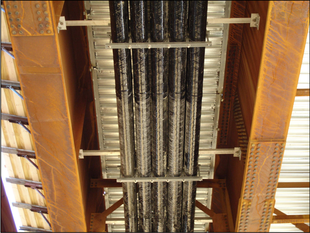
Example of Typical Fiber Installations Within Existing Bridge Conduit
