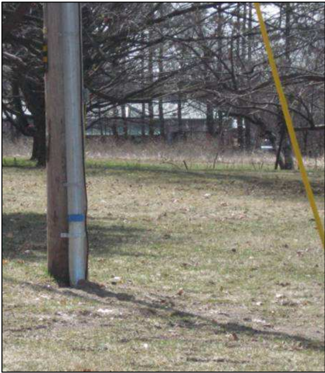
Typical Fiber Installation. The figures above (provided by Fibertech) show how new cable would be run underground using existing conduit. Generally, the aerial fiber runs down the pole and then routes inside the existing conduit that is located next to the pole.
