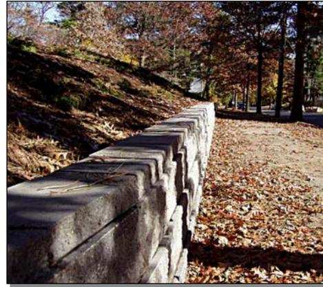
deep and weigh 81 pounds each! The block used is the Diamond Pro series straight face type with a "gray flash" color ( a blend of charcoal and natural color) made by Grinnell.
