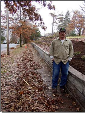
spread the last load of bark mulch the week of November 13<sup>th</sup>. The final dimensions of the wall are 250 linear feet with a height of two feet. Three courses of blocks and one course of
