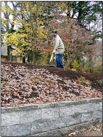
capstones are what give the wall its height. The wall consists of 480 wall blocks and 200 capstones. The wall blocks measure 8" high, 18" long, are 12"
