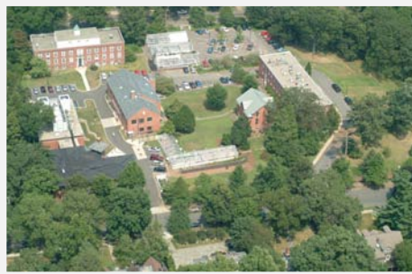
Main Laboratories, New Haven
