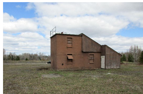
The Burn House at the former Loring Airforce Base.
