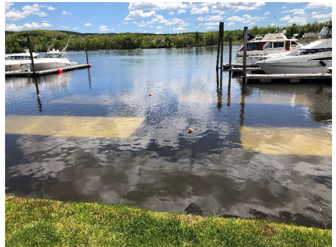
Benthic barriers installed at Portland Boat Works.
