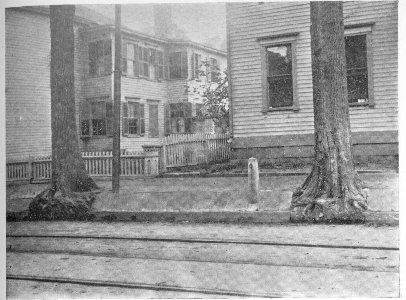
Fig. 3. —Trees mutilated in laying curb and gutter.
