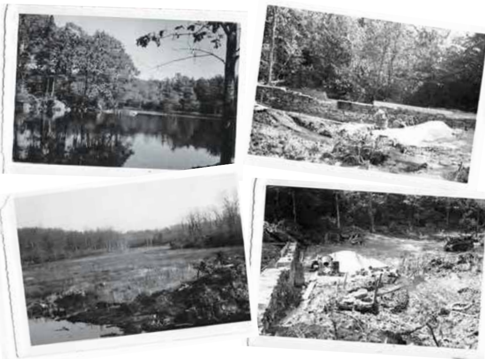
Snapshots show progress in the building of the dam for the pond in the 1950s. Photos courtesy of Marge McIntosh
