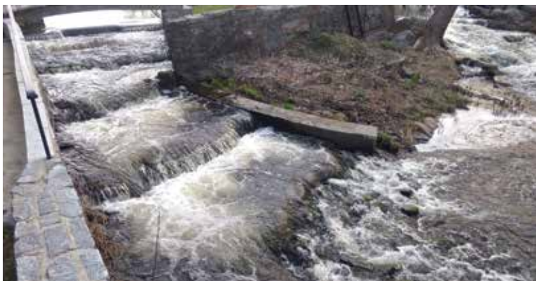
The Tiley-Pratt Dam on the Falls River in Essex is an example of a dam not listed as a priority in 1962, but a fishway was built in 2017 at this private home to restore the run of alewives.
