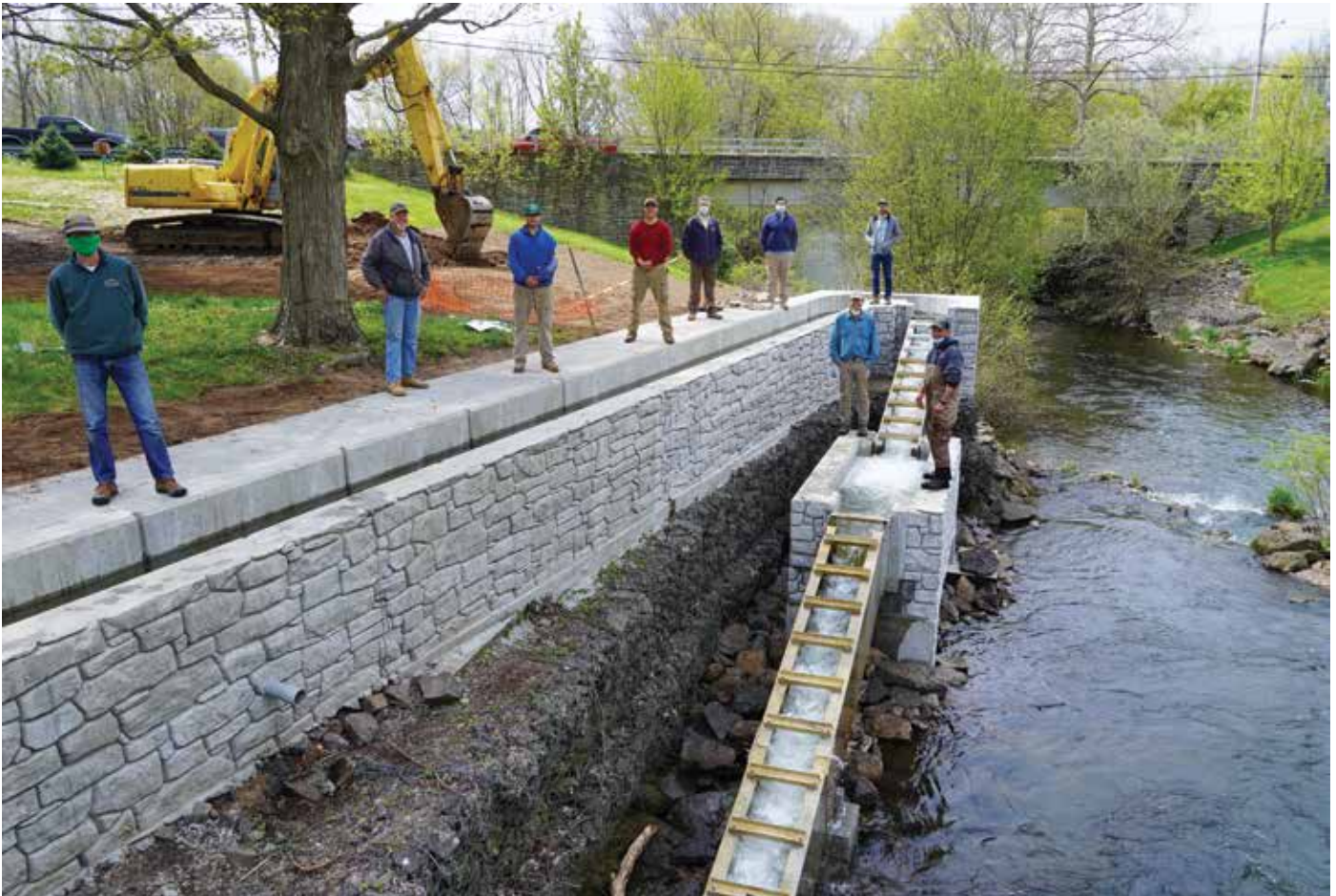
Pages Millpond Dam in North Branford is the second dam on the Farm River (#27 in the table) and its steepass fishway was completed in 2020, 58 years after the State Board of Fisheries and Game report recommended it. Like many fishways, this is on private property but can be seen from the Mill Road Bridge.
