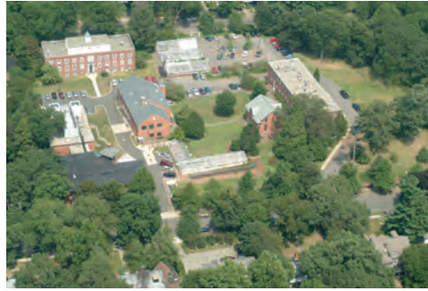
Main Laboratories, New Haven
