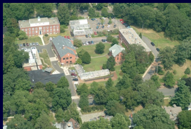
Main Laboratories, New Haven
