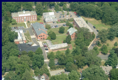
Main Laboratories, New Haven
