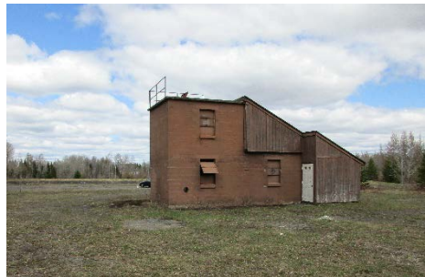
The Burn House at the former Loring Airforce Base.
