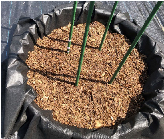
Figure 6. Pool with 2" of pine bark mulch drainage layer installed.
