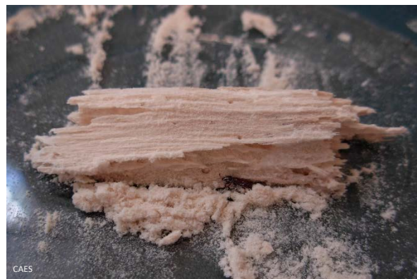
Fig. 2: Powderpost beetle damage
