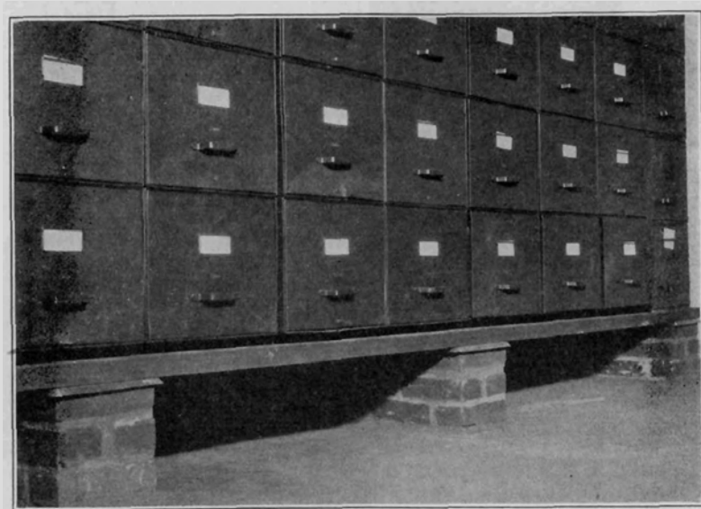
FIGURE 89. Records stored on termite-proof rack in basement of an infested building.
